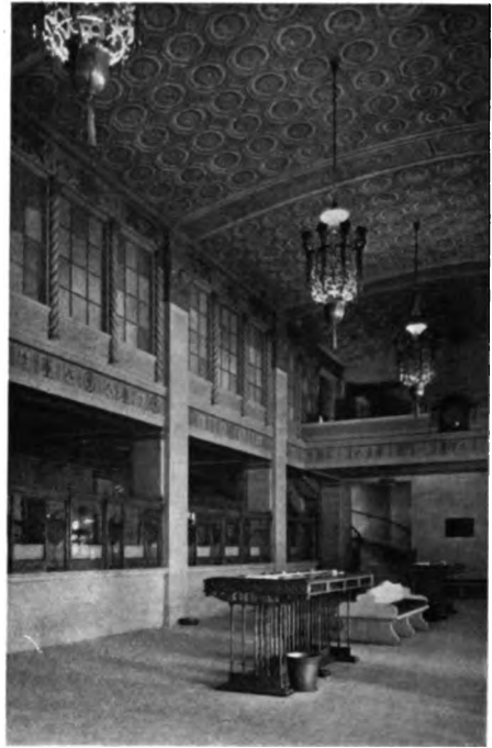
Corner of banking room looking toward stairway to mezzanine
