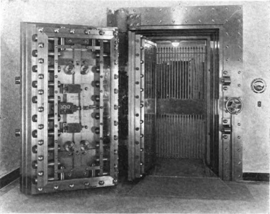
The great doors to the vault, showing the intricate work and massive locking bolts, 24 in number This huge vault contains space for over 10,000 individual safe deposit boxes
