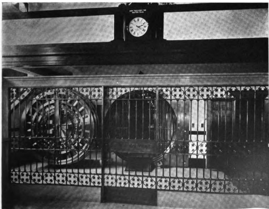
Safety deposit vault
