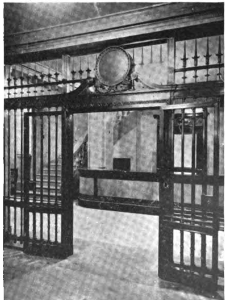
Grilled entrance to the safe deposit vaults
