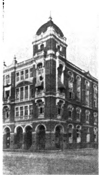
The Central Bank of India, Ltd., Hornby Road, Bombay
