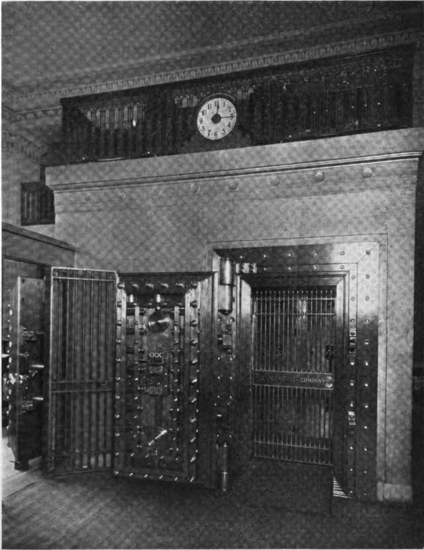
Entrance to the safe deposit vault
