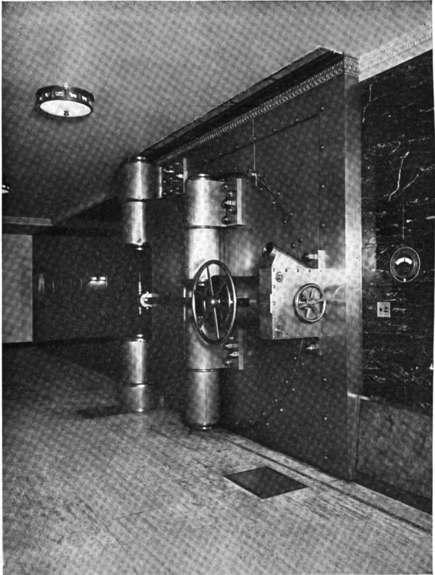
VIEW OF MASSIVE DOOR CLOSED
