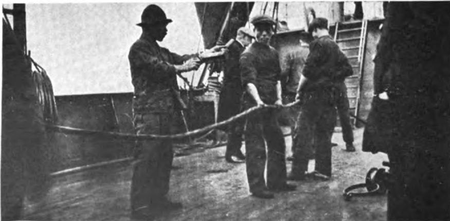
Splicing a broken cable before "paying" overboard
