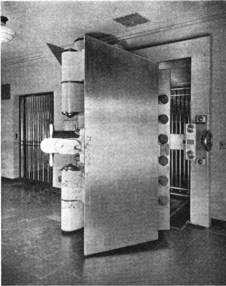
Rectangular vault door 36 inches thick, built by York Safe & Lock Co. for new Bowery Savings Bank vault
