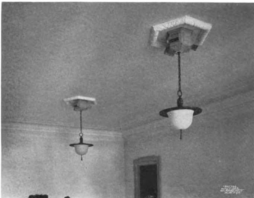
Ceiling of the council room, London, Liverpool & Globe Insurance Co., New York. Two ceiling outlet boxes are shown in this illustration, each fitted with three swivel nozzles. The lighting fixtures are a part of the same units
