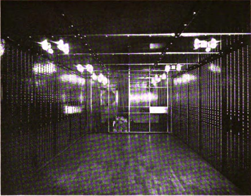
Interior of safe deposit vault having capacity for 8,000 boxes. The vault has heavy steel lining with two feet of concrete reinforcing
