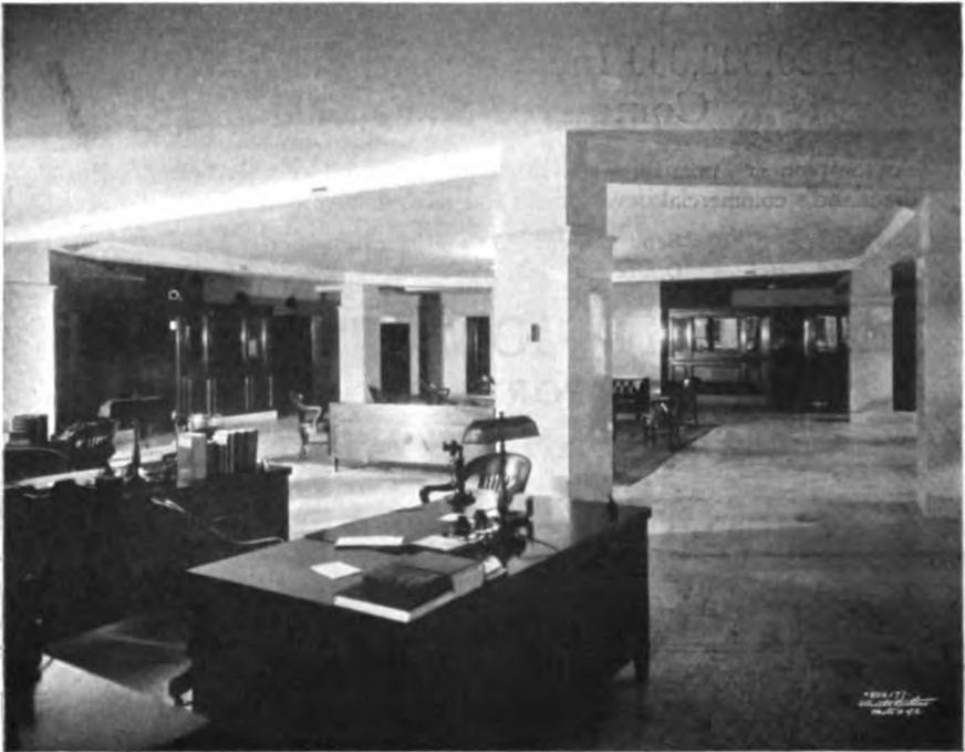
A section of the officers' quarters, Seaboard National Bank, New York, showing distributing air ducts which are at the ceiling between the interior columns and which have the appearance of ceiling beams. The nozzles or air outlets are on the side of the ducts
