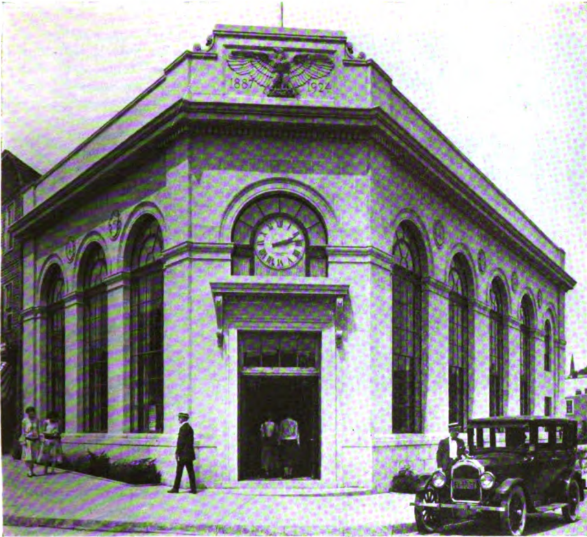
Exterior of the Union Savings Bank of Westchester County, Mamaroneck, N. Y.
