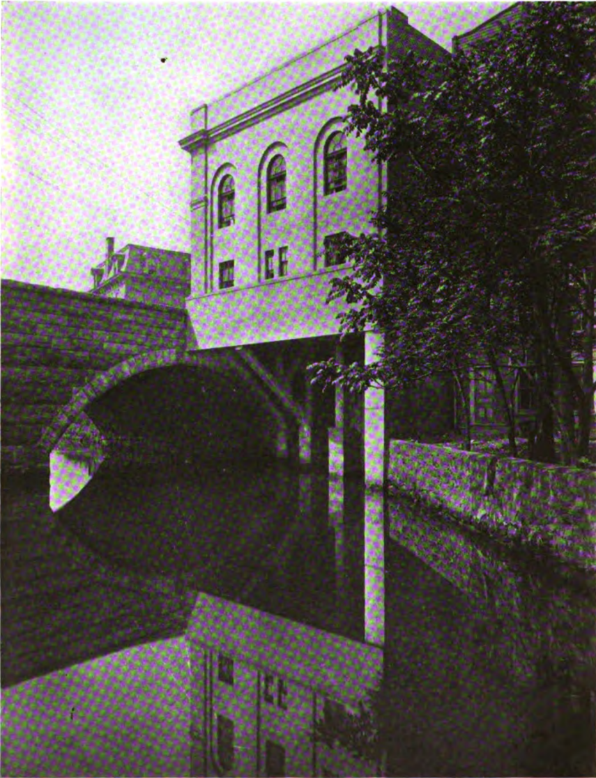
A view of the rear of the Union Savings Bank of Westchester County, Mamaroneck, N. Y., showing how the bank overhangs a stream without having any vertical supports in the stream. The building was planned and erected under the supervision of Morgan, French & Co., Inc., architects and bank engineers, New York
