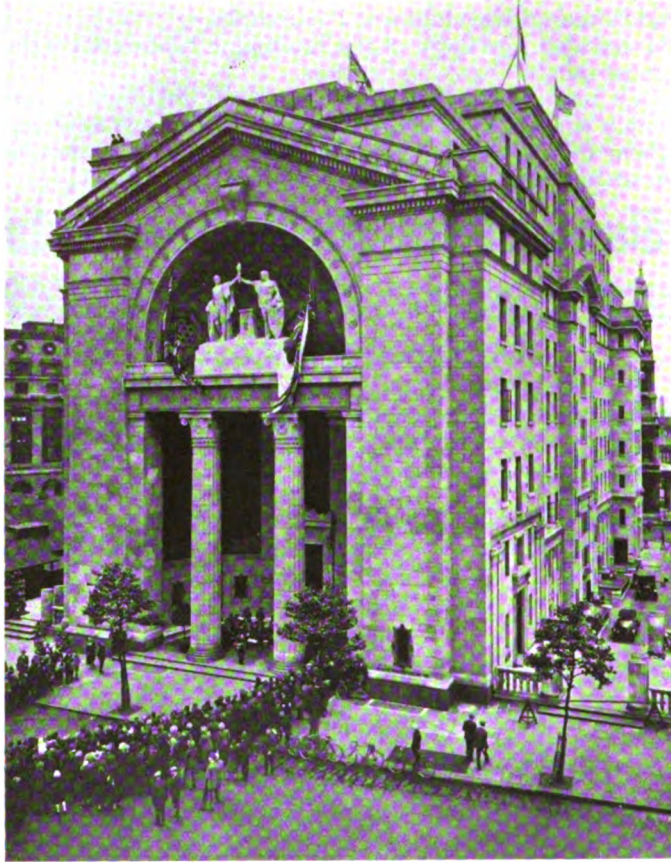
Bush House, London, the building shown above, was formally opened on July 4, with addresses by Earl Balfour and Irving T. Bush. It is intended as a memorial of the friendship between the English speaking peoples. The building was designed by Helmle and Corbett, London, and the sculpture group above the entrance is the work of Malvina Hoffman of New York
