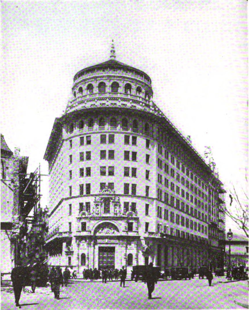
The new building of The First National Bank of Boston, Buenos Aires branch. The building was designed by Chambers & Thomas of Buenos Aires, with York & Sawyer of New York as consulting architects. It was constructed under the supervision of Stone & Webster, Inc., of Boston
