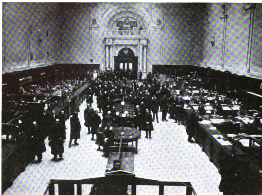
Main banking floor of the Bank of Poland
