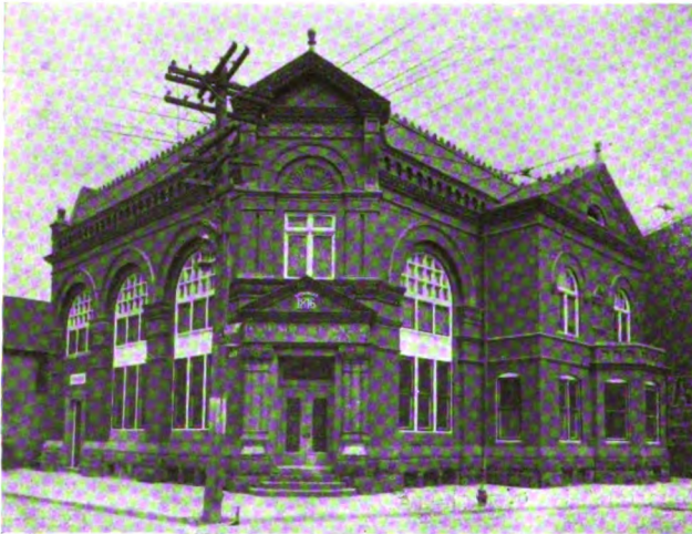
Exterior of the Cumberland National Bank, Bridgeton, N. J., after recent alteration.
