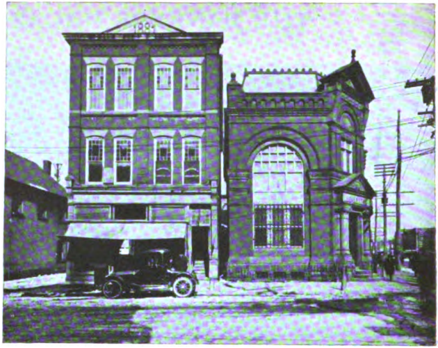
Exterior of the Cumberland National Bank before recent alterations by the Griswold Building Company, Inc., New York, specialists in bank building and designing.
