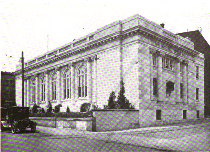
The Bristol Trust Company, Bristol, Conn., as seen from the rear, after completion of alterations and additions by the Griswold Building Co., Inc., New York
