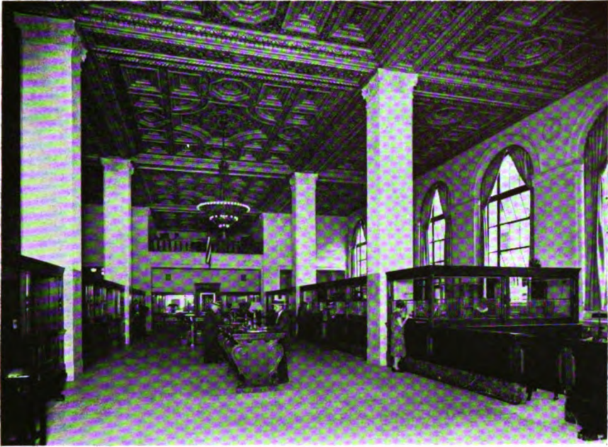
Main Banking Room Trenton Trust Company, Trenton, N. J.
