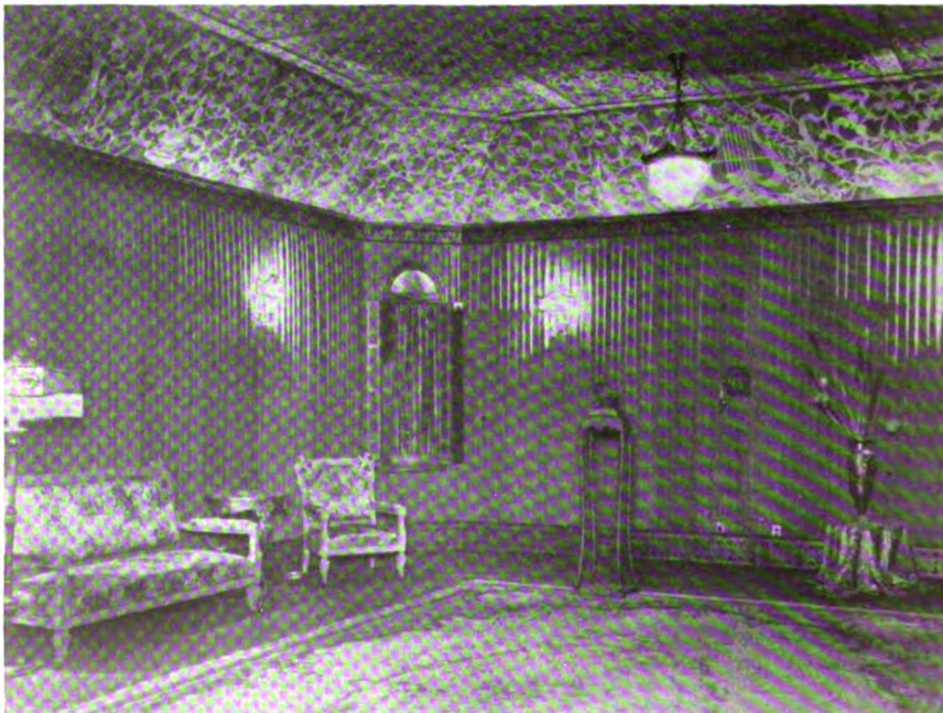
Radio station KFVB, Los Angeles, Calif., owned by Warner Bros. Celotex, decorated, used for acoustical correction.
