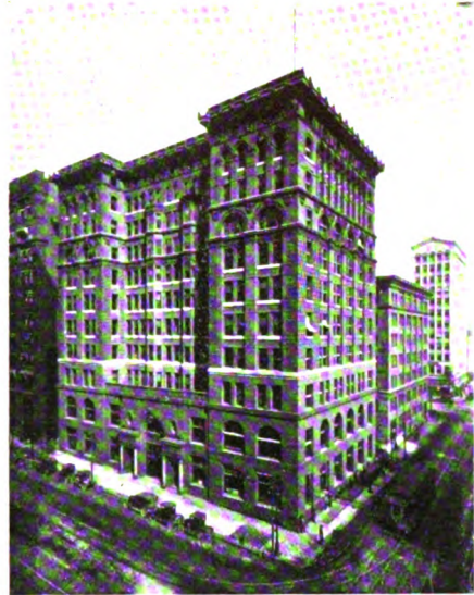
The Union Trust building, recently purchased by the Fidelity Trust Co., of Detroit.
