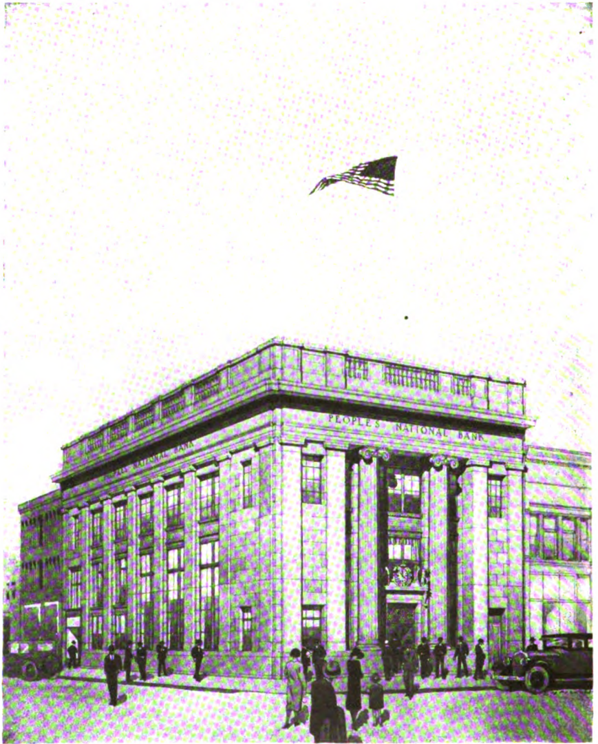
PEOPLES NATIONAL BANK LATROBE, PENNA. (UNDER CONSTRUCTION)
