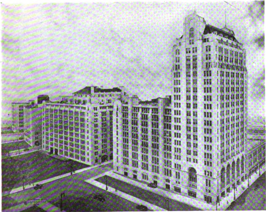
Santa Fe Terminal building, Dallas.
