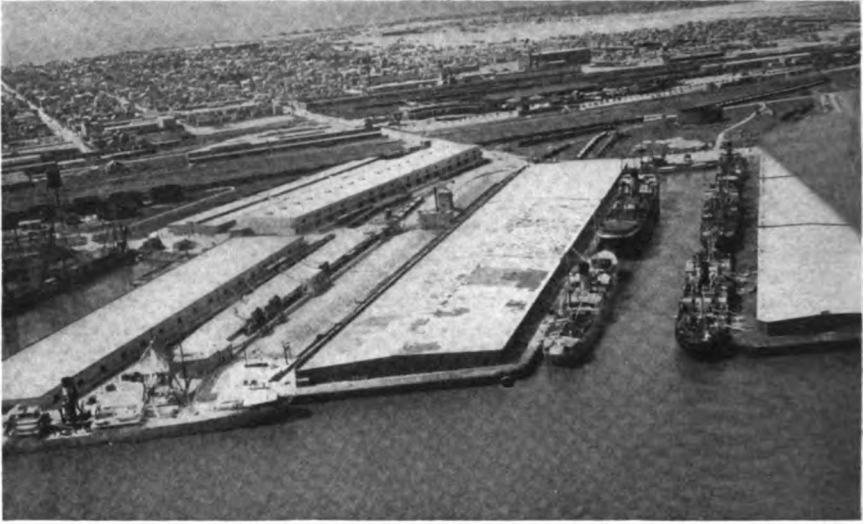
A portion of Galveston's waterfront, showing the dock where more than 600,000 tons of sulphur were loaded into ships during 1925. Note how the slip system is followed out.
