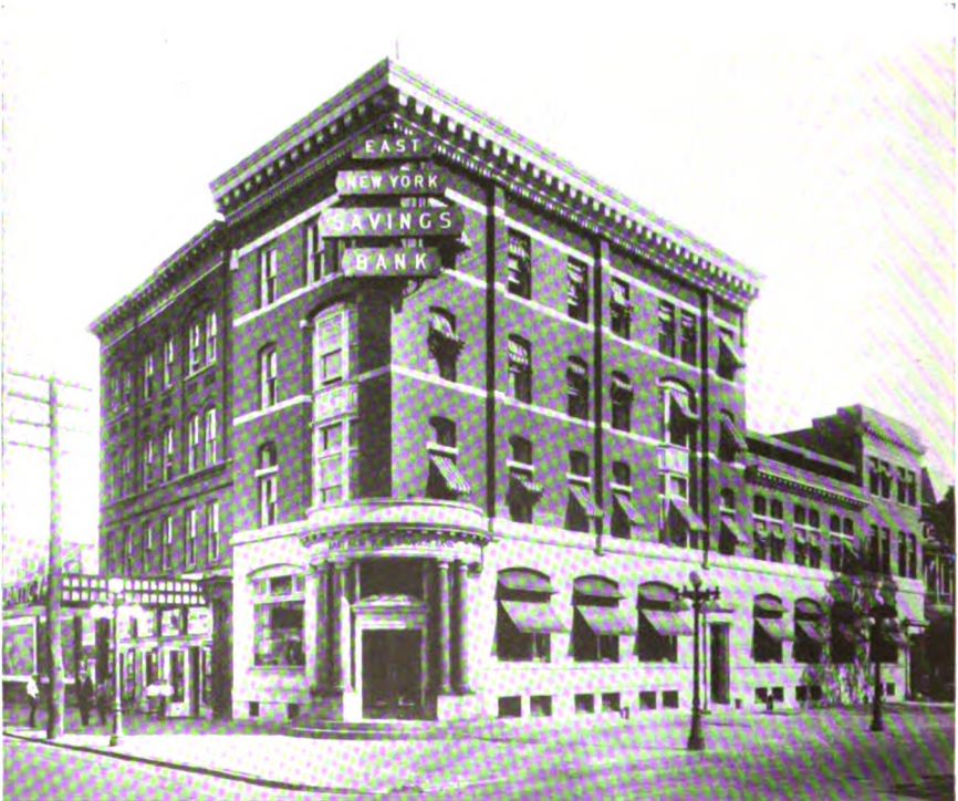
Exterior of the newly altered and enlarged East New York Savings Bank, Brooklyn, N. Y., showing addition at the rear and the first floor refaced with limestone. The interior was also modernized and a large safe deposit department provided for in the basement. The remodelling was the work of Holmes and Winslow, architects, New York City.
