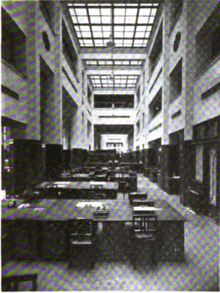
Interior view of main office.
