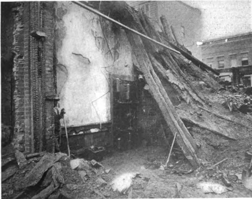
The fire-resisting qualities of the modern bank vault were illustrated in a recent fire which completely demolished the Farmers National Bank of Hudson, N. Y. The vault, pictured above, was undamaged on the exterior except for the outside finish and the rubber grips on the spokes of the wheel, which grips were melted off in the fire. The interior was found to be in first class condition, when the vault was opened after it had cooled off, a few days after the fire. The vault was installed a few years ago by the York Safe and Lock Company, York, Pa.
