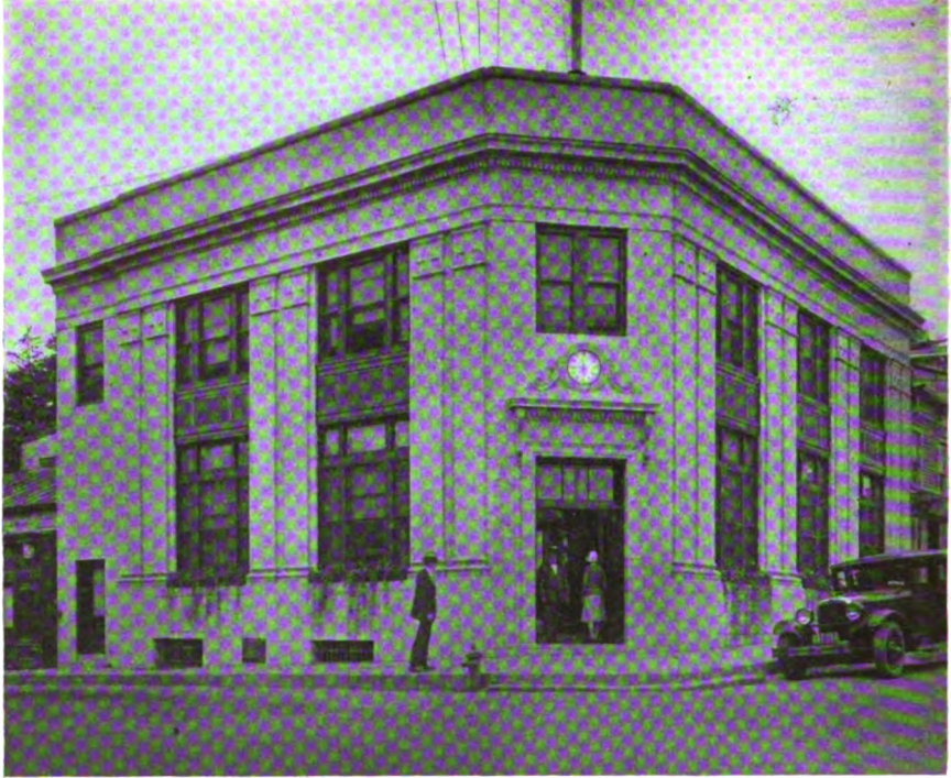
Remodeled building of the First National Bank, Marlborough, N. Y. This building was recently remodeled and extended with a complete new front in Indiana limestone and with new banking equipment under the supervision of Morgan, French & Co., architects and engineers, New York.
