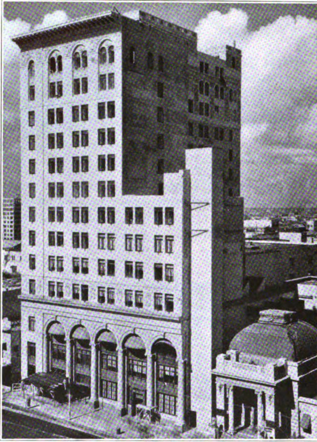
THE FIRST UNIT OF THE 13-STORY BANK AND OFFICE BUILDING FOR THE BANK OF BAY BISCAVNE, MIAMI, FLA.
