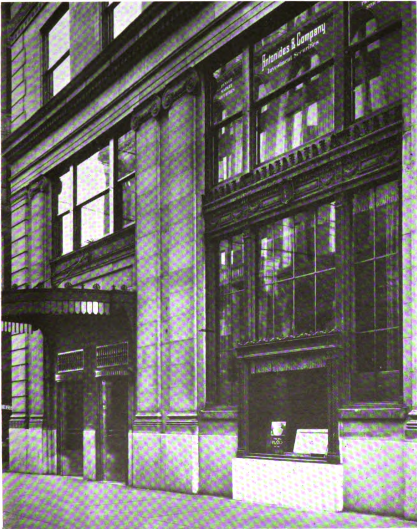
The United States National Bank of Denver, Colo., has solved the problem of installing a display window in a bank building whose present windows have high sills, as shown above. The exterior of the window is of cast metal and glass and the interior of walnut.
