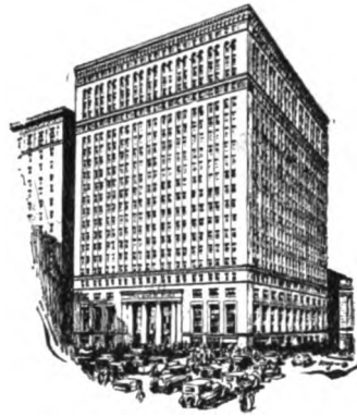
New Home of the State Bank of Chicago — now being erected at La Salle and Monroe Streets, the center of Chicago's financial district.
