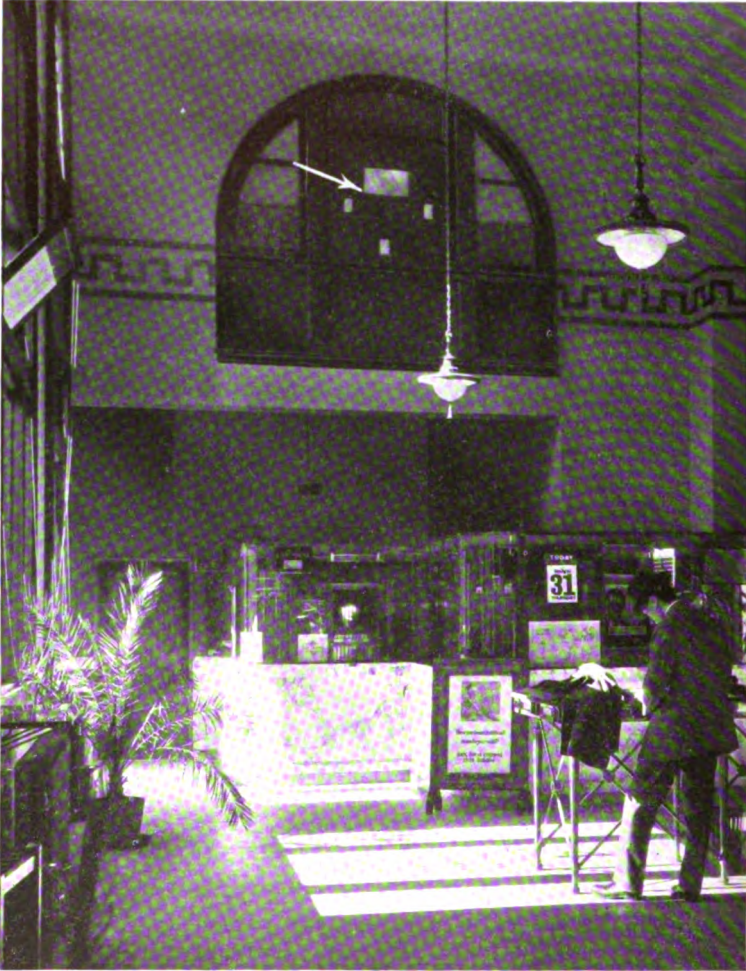
Lobby of Elizabethport Banking Company. Arrow in upper background indicates observation window and firing apertures in bullet proof steel compartment on mezzanine floor in rear of bank. Any part of lobby can be instantly brought under fire by guard in cage.
