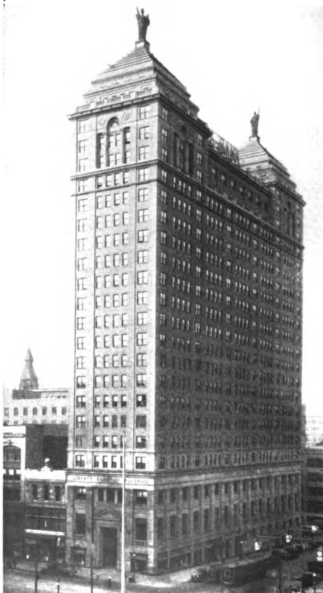
The new home of the Liberty Bank of Buffalo, Buffalo, N. Y., not only furnishes the bank with modern and adequate banking quarters, but provides an excellent office building as well. The building was designed by Alfred C. Bossom, bank architect and equipment engineer, New York.
