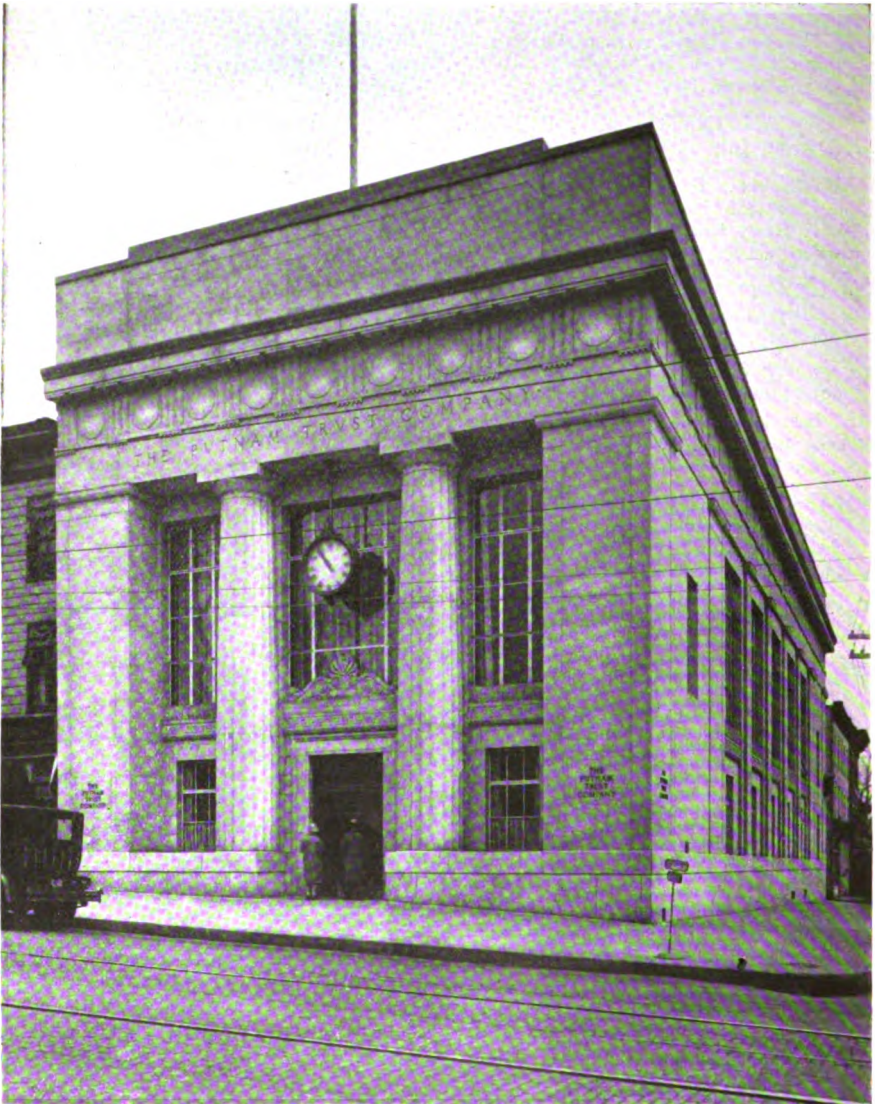
The new home of the Putnam Trust Company, Greenwich, Conn., is of Indiana limestone and of Greek Doric design. The building and its equipment were designed by and erected under the supervision of Morgan, French & Co., Inc., architects and engineers of New York.
