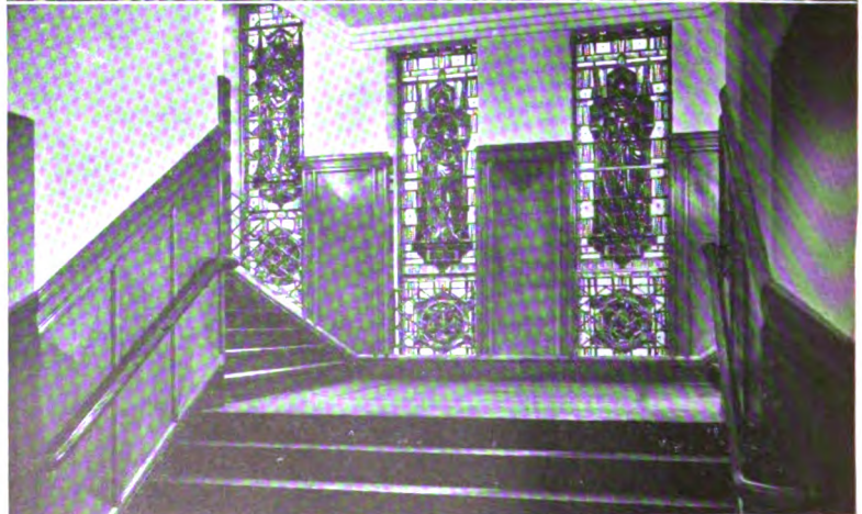
Stairway to main floor.
