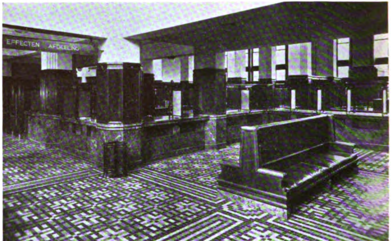
Partial view of main banking room.
