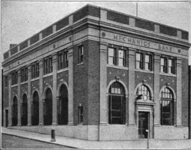
The Bay Ridge branch of the Mechanics Bank, Fourth avenue at 51st street, Brooklyn, New York, is of light buff brick of a rough texture, with cast iron trim. The ground floor and mezzanine are occupied by the bank, while the upper floor is rented. The building was designed by Holmes & Winslow, bank architects, New York.
