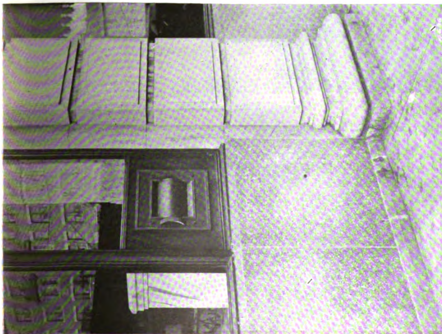
Two views of the night depository equipment of the Chelsea National Bank, Atlantic City, N. J. At the left is the exterior rotary receiving station which the depositor has a key and into which he places his deposit, previously locked in a canvas bag. At the right is the interior receiving chest into which the deposit falls and where it remains until opened by bank officials. The difficulty of installation in this case was overcome by cutting down a window and installing a bronze panel thereon. It is possible to install the depository under almost any conditions. The vault was designed and installed by the Bank Vault Inspection Company, Philadelphia.
