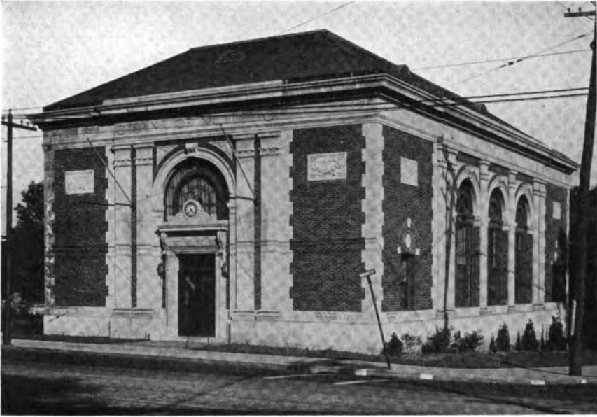
The Colonial building of the Bank of Nutley, Nutley, N. J., is of red tapestry brick, with a base of Woodbury granite. Pilasters and cornices, etc., are of Bedford limestone and the roof is of slate shingles in various shades.
