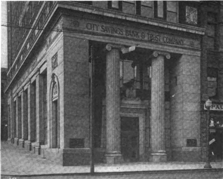
Bank and Office Building for City Savings Bank and Trust Company, Alliance, Ohio Designed by and erected under the supervision of SIMONS, BRITTAIN & ENGLISH
