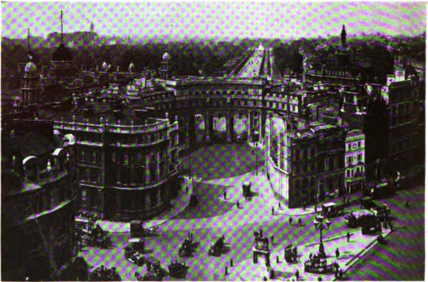
View showing Drummonds' branch (on left of Admiralty Arch) at Charing Cross.
