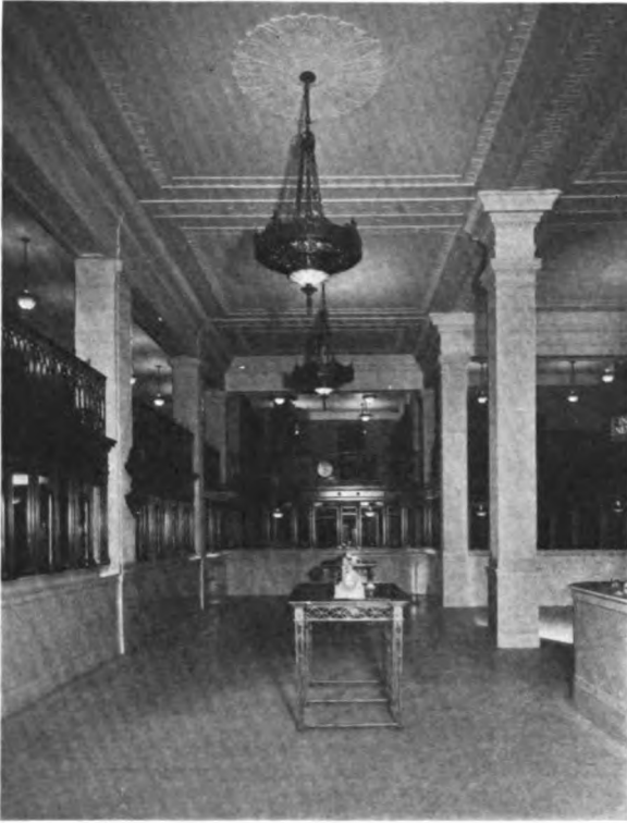
View of the main lobby (left) of the Franklin Society for Savings, New York, which has recently moved into new quarters at 217 Broadway. The officers' quarters are shown below.
