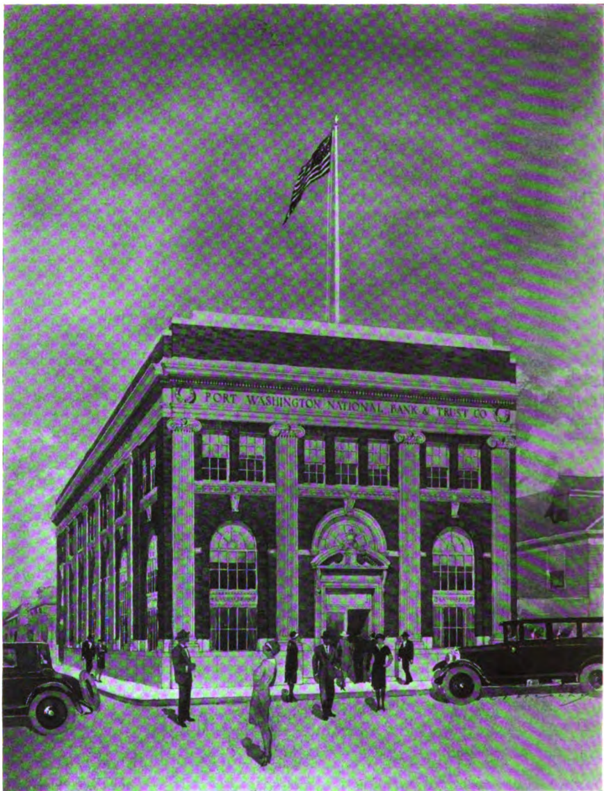
PORT WASHINGTON NATIONAL BANK & TRUST CO., PORT WASHINGTON, N. Y. (UNDER CONSTRUCTION)
