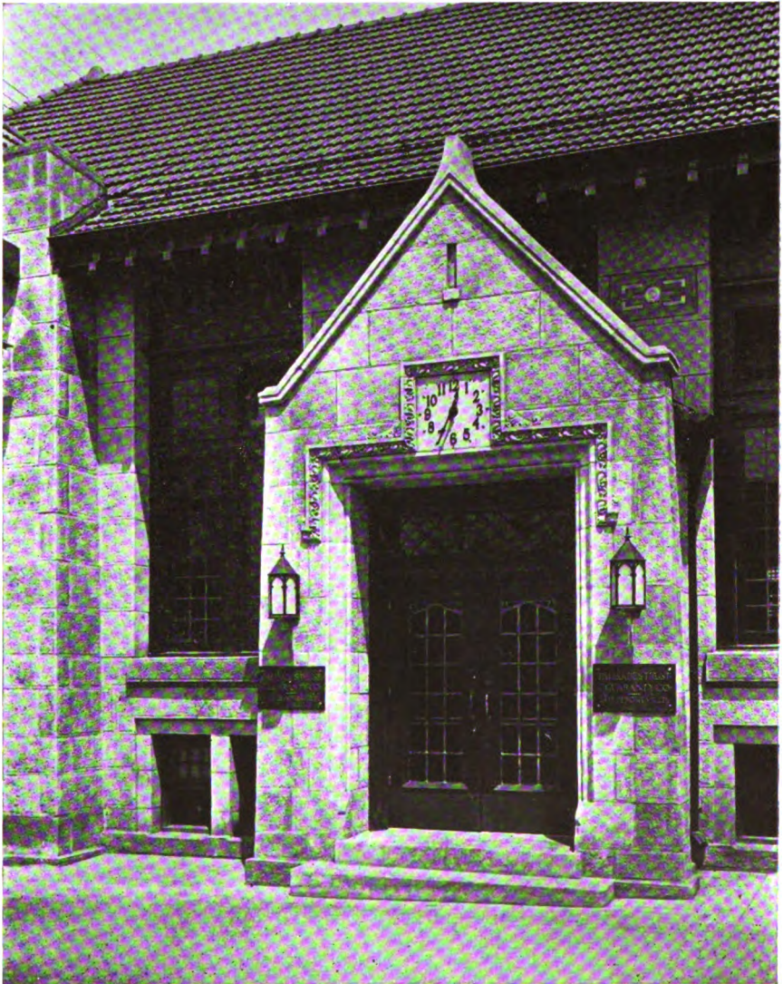
This interesting and unusual type of main entrance is the result of the remodelling of the old entrance of the Palisade Trust and Guaranty Company, Englewood, N. J. The entire old building was left standing while a new entrance and additions to sides and rear of the building were constructed. Holmes & Winslow, specialists in bank architecture, New York City, were the architects.
