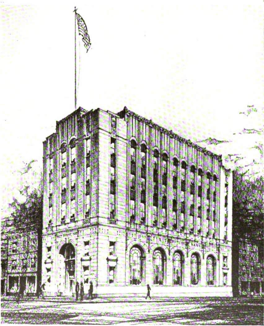
Indiana limestone, enriched by polished granite columns, lends dignity to the First National Bank, Carbondale, Pa., being built by Tilghman Moyer Company, architects and engineers, Allentown, Pa.
