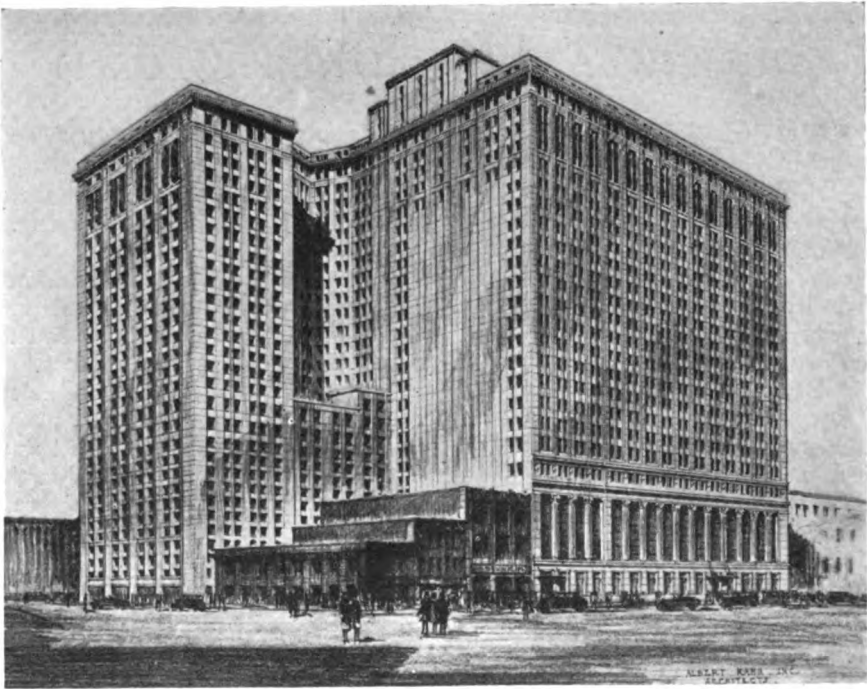
First National Bank in Detroit, Mich., as it will look after the new twenty-five story addition is completed.
