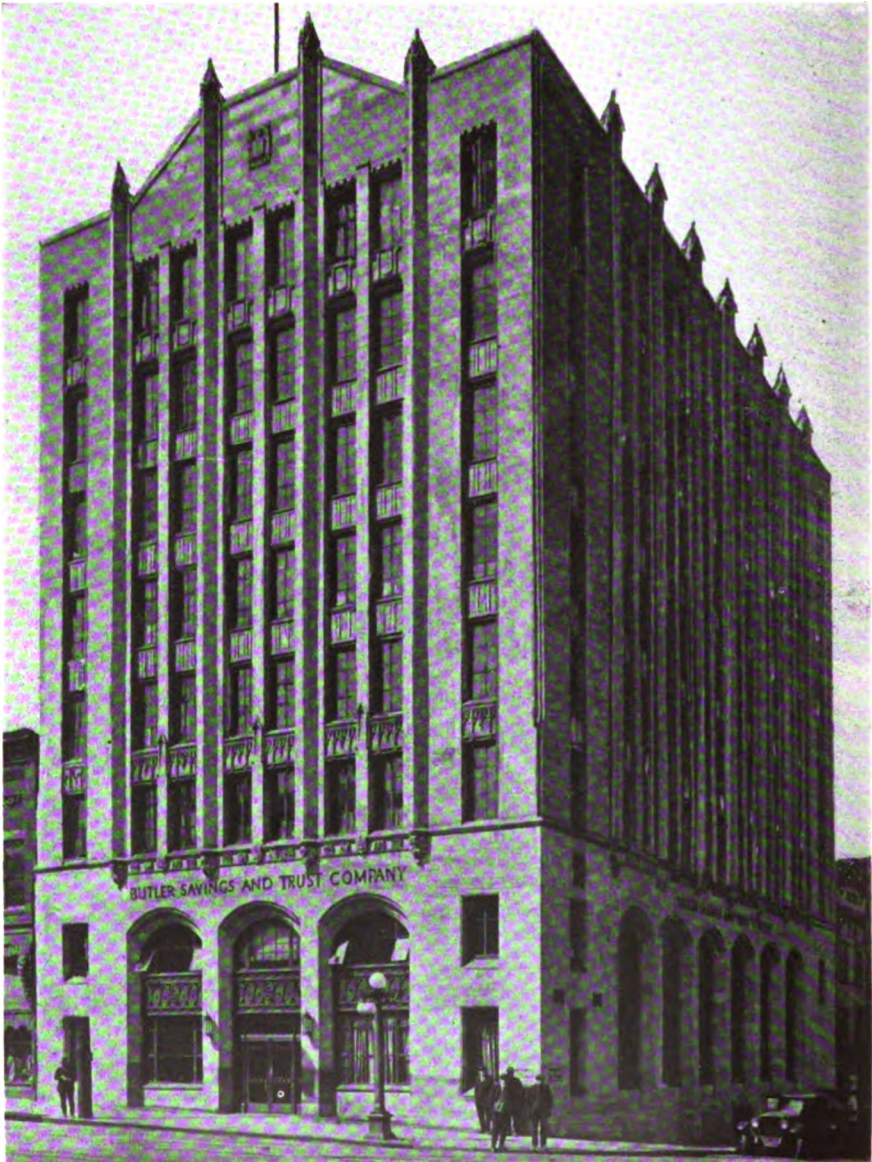
The building of the Butler Savings & Trust Company, Butler, Pa., was designed to make more prominent the name of the bank and to provide the most modern banking facilities. It stands on a site 60 by 105 feet. The exterior is of Indiana limestone and the entire building is of fireproof construction. Uffinger, Foster & Bookwalter, Inc., New York, designed the building and supervised its erection.
