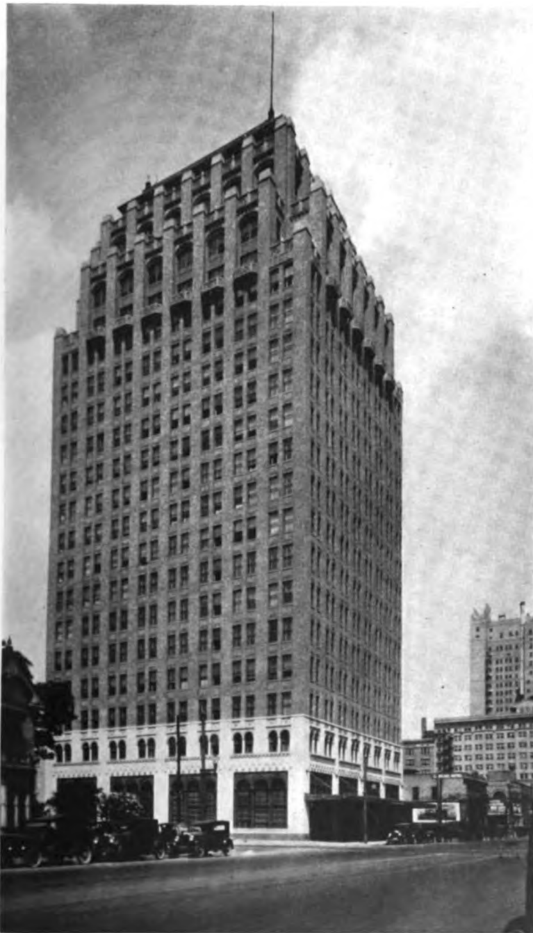
The Petroleum building, a twenty-one story office building, is the home of the Fidelity Trust Company of Houston, Texas. The building is of the modern recessional type and its detail was inspired by the architecture of the Mayan Indians in Yucatan, Central America. The base is of Indiana limestone and the shaft and upper portion of brick trimmed with terra cotta. The building was designed by Alfred C. Bossom, bank architect and equipment engineer, New York.
