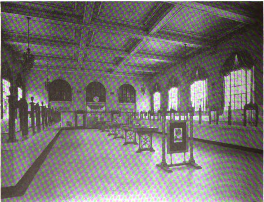
Interior view of the new building of the Des Plaines State Bank, Des Plaines, Ill. The vault installation was made by the York Safe & Lock Company, York, Pa.
