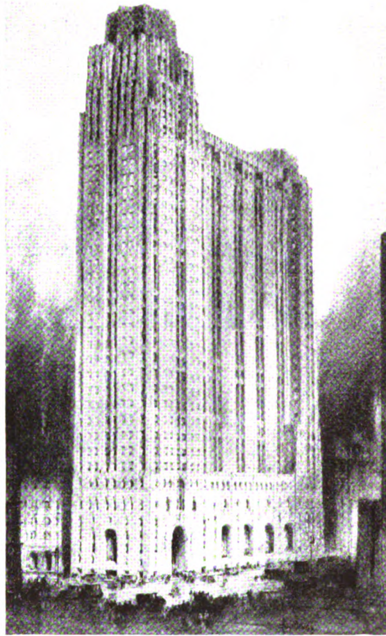
New Union Trust Building, Detroit, now under construction
