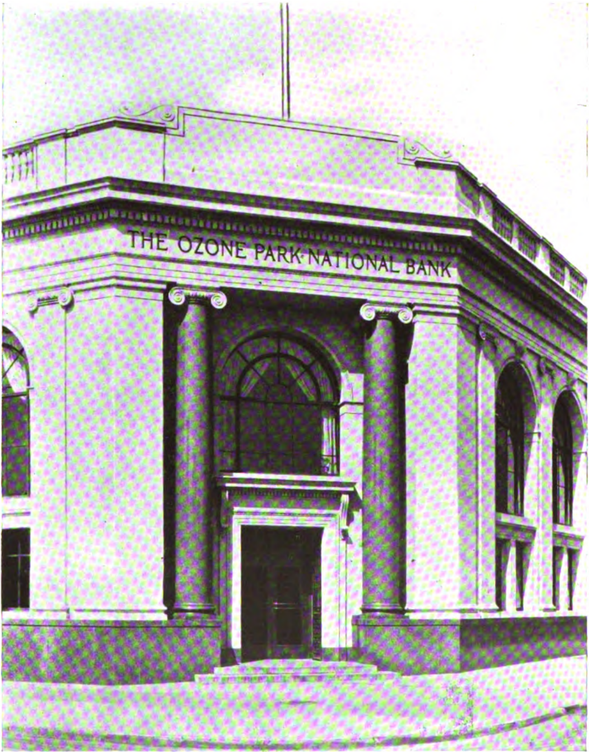
The exterior walls of the new Ozone Park National Bank, Ozone Park, Long Island, N. Y., are of cast stone in imitation of light gray granite. The base is of polished green granite and the columns at the entrance are monoliths of the same stone. The window and entrance door frames are of bronze, and the corner entrance is at the intersection of two important thoroughfares. Uffinger, Foster & Bookwalter of New York were the designers and supervisors of the building.
