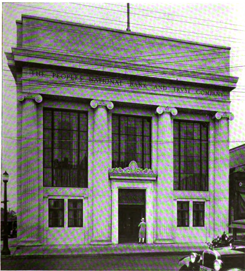
The new, individual building of the Peoples National Bank and Trust Company, Lynbrook, Long Island, N. Y., is of Indiana limestone with granite base, the front having a massive colonnade in Ionic style. The same classic treatment is carried out on the sides of the building, with pilasters between which are large windows. The windows are metal, of modern type and the entrance doorway is of bronze. The building was designed by and constructed under the supervision of Morgan, French & Co., Inc., architects and engineers, New York City.
