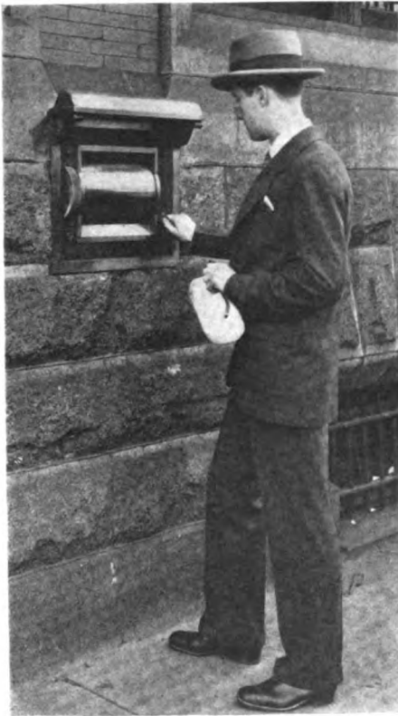
ROTARY WITH FLOOD LIGHT AT THE NORTHERN NATIONAL BANK, PHILADELPHIA
