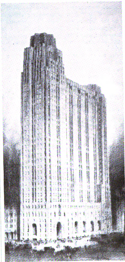
New Union Trust Building, Detroit, now under construction
