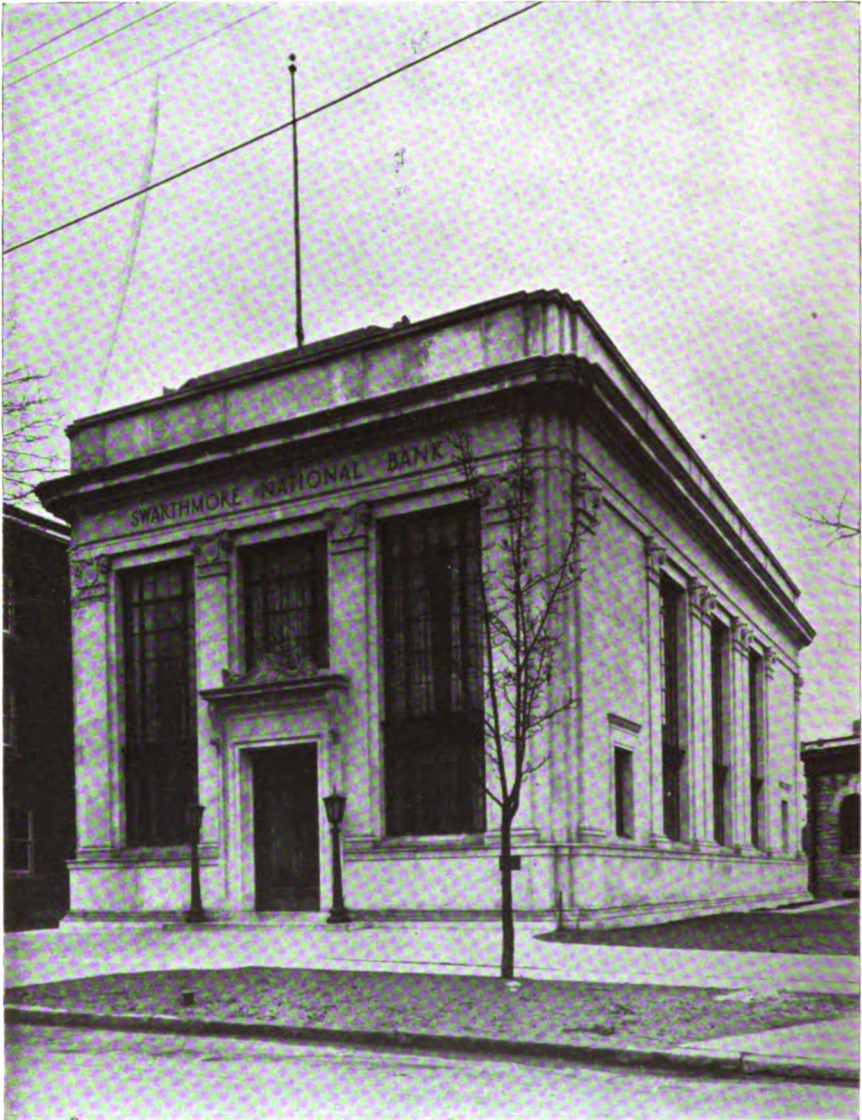
Indiana limestone again proves its excellence in the quiet dignity of the Swarthmore National Bank, Swarthmore, Pa., designed, constructed and furnished by the Tilghman Moyer Company, Allentown, Pa. The windows are of a special design executed in steel.
