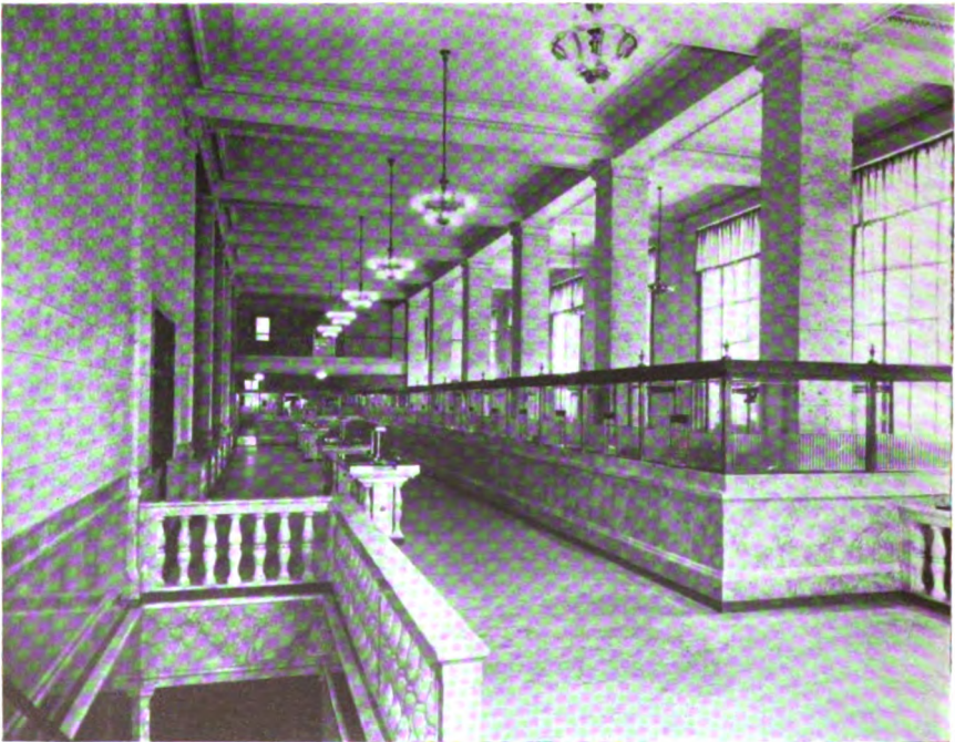
The stairway at the left of the main banking room of the Globe Exchange Bank, Brooklyn, N. Y., leads to large foreign, trust and safe deposit departments in the basement. Uffinger, Foster & Bookwalter, New York, were the architects.
