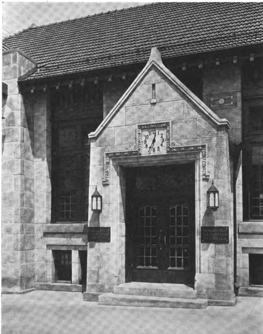
Remodelled Main Entrance of the Palisade Trust and Guaranty Company, Englewood, N. J.
