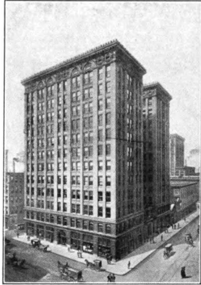
LINCOLN TRUST COMPANY BUILDING.
