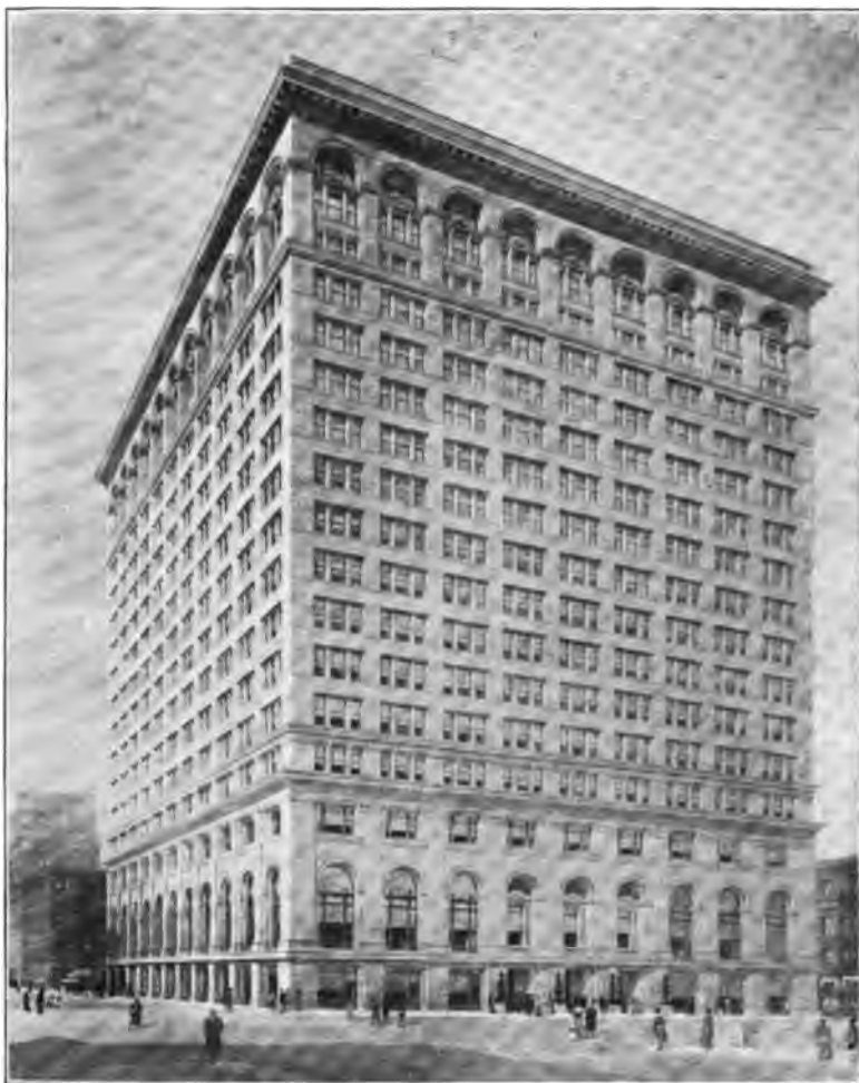
NEW BUILDING BEING ERECTED BY THE FIRST NATIONAL BANK OF CHICAGO.
