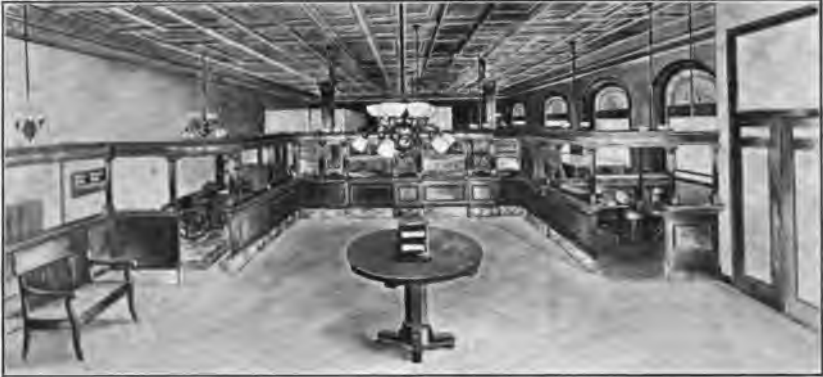
MERIDIAN NATIONAL BANK—INTERIOR VIEW.
