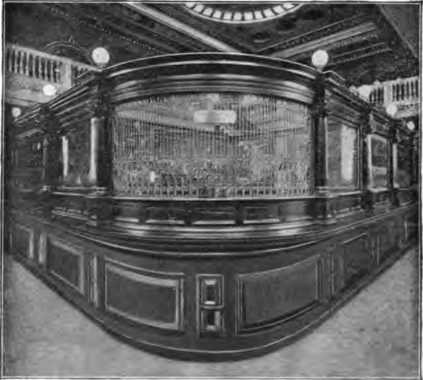
INTERIOR VIEW OF THE CORN EXCHANGE NATIONAL BANK.
