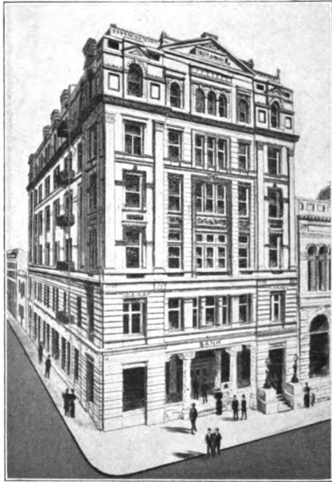
SAN FRANCISCO SAVINGS UNION. Building destroyed. Temporary office, 2617 Pacific Avenue.
