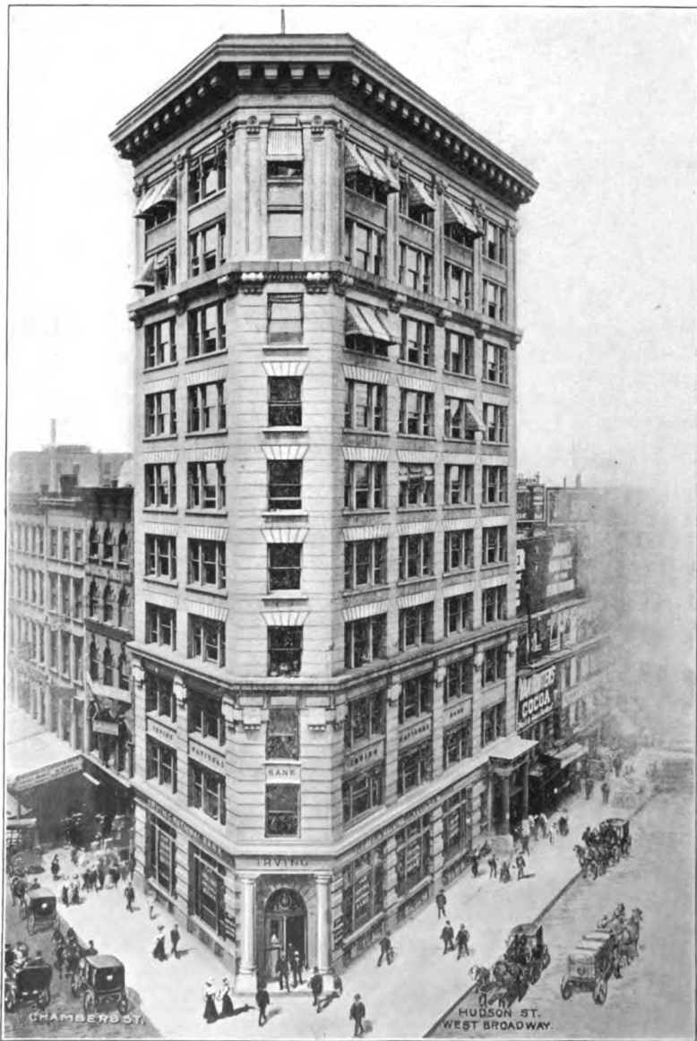
IRVING NATIONAL BANK BUILDING, NEW YORK.
