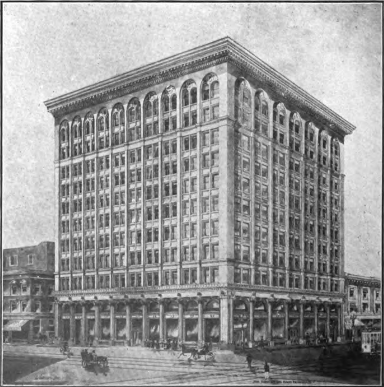
SECURITY SAVINGS BANK BUILDING, (Under Construction.)
