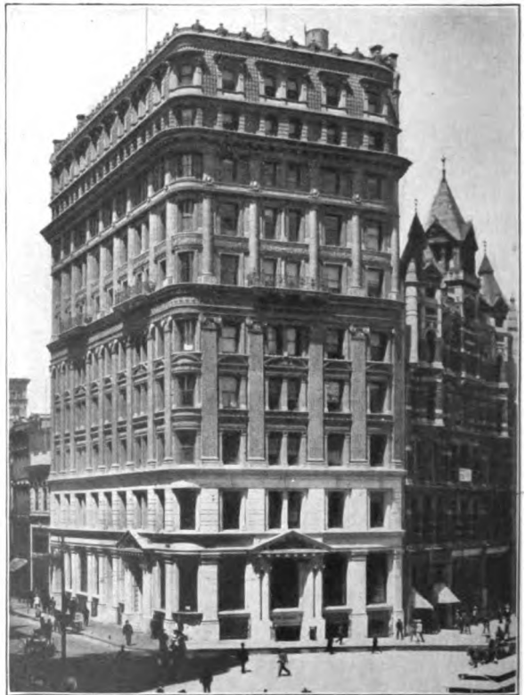
UNION TRUST COMPANY. Building damaged, but available for use.
