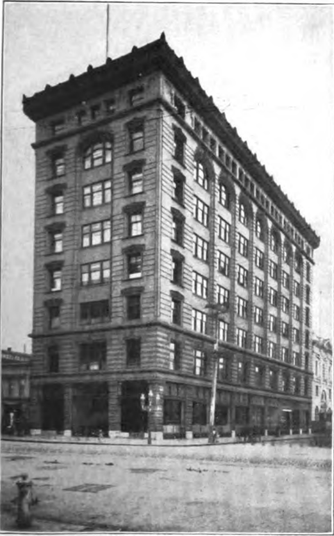
THE MARKET STREET BANK. Building damaged, but available for use.
