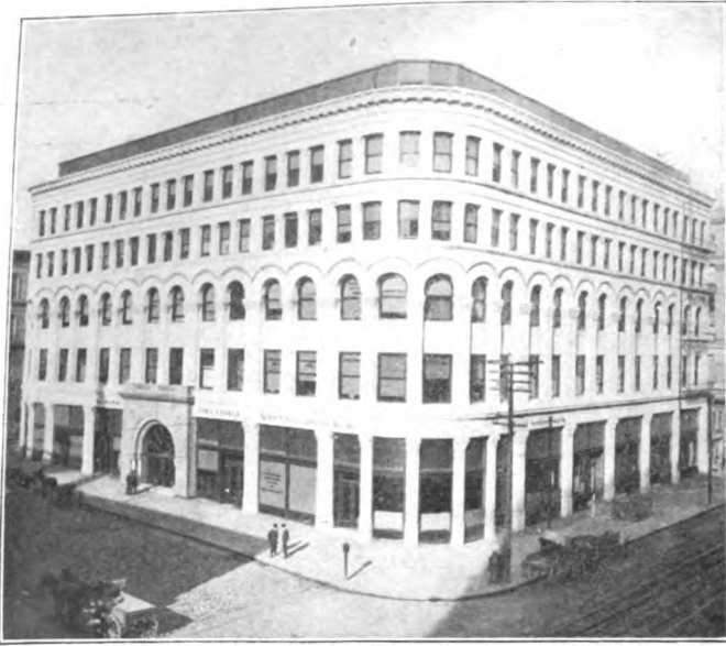
GERMANIA NATIONAL BANK. Building destroyed. Temporary office, 214 Laguna Street.
