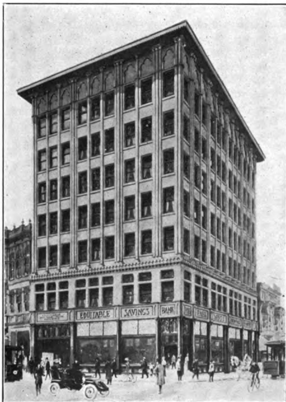
EQUITABLE SAVINGS BANK. (Under Construction.)
