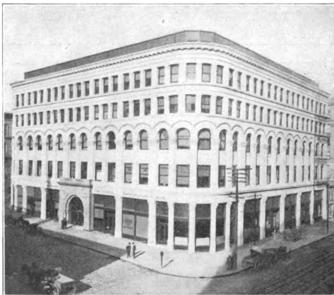
GERMANIA NATIONAL BANK. Building destroyed. Temporary office, 214 Laguna Street.
