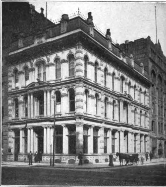
ANGLO-CALIFORNIAN BANK, LIMITED. Building destroyed. Temporary office, southwest corner Clay and Franklin Streets.
