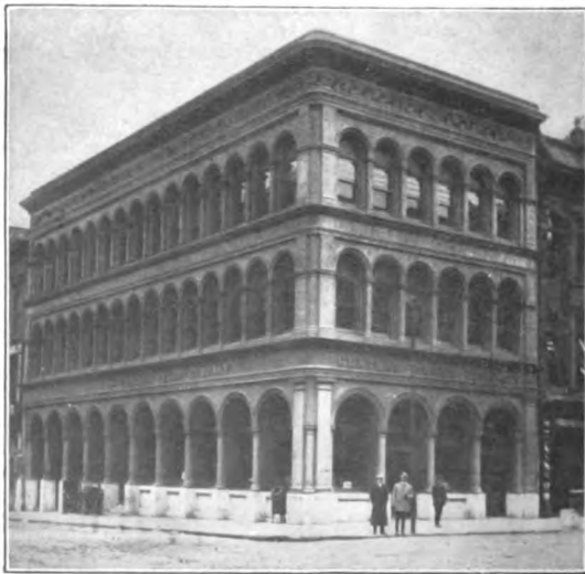
CENTRAL TRUST COMPANY. Building destroyed. Temporary office, 2121 Laguna Street.
