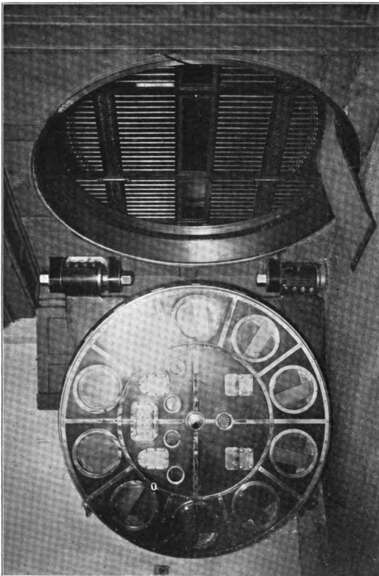
MANGANESE VAULT CONSTRUCTED FOR HARVEY FISK & SONS, NEW YORK CITY. Dimensions, 9' x 9' x 13' 8".
