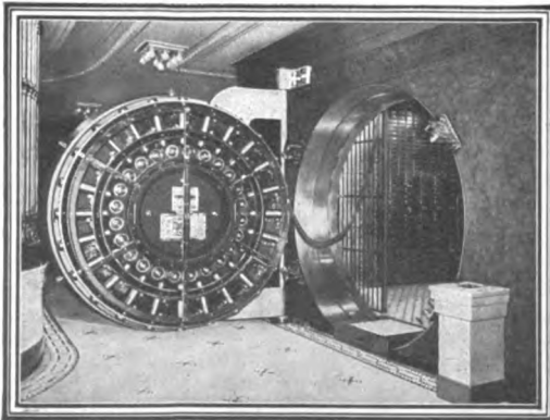
Entrance and Door to Vault.
