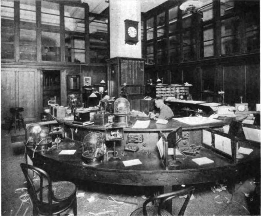
The Wire Room.
