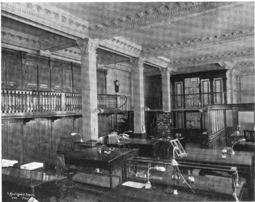
Working Quarters of the Banco Oriental de Mexico, S. A.
