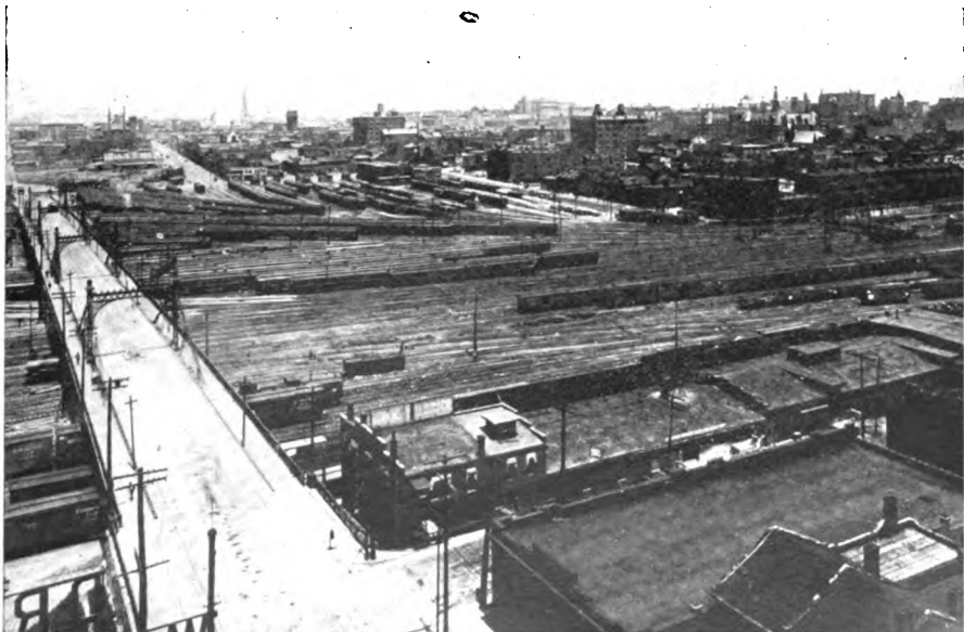
Mill Creek Valley, St. Louis, showing tracks leading from the Union Station—a feature of the Terminal System.
