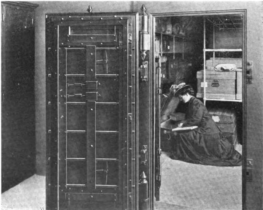
One of the Storage Vaults.
