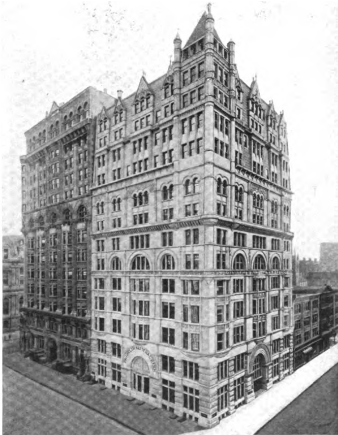
Modern Sky-Scraper Home of the Franklin National Bank of Philadelphia, at Broad and Chestnut Streets.
