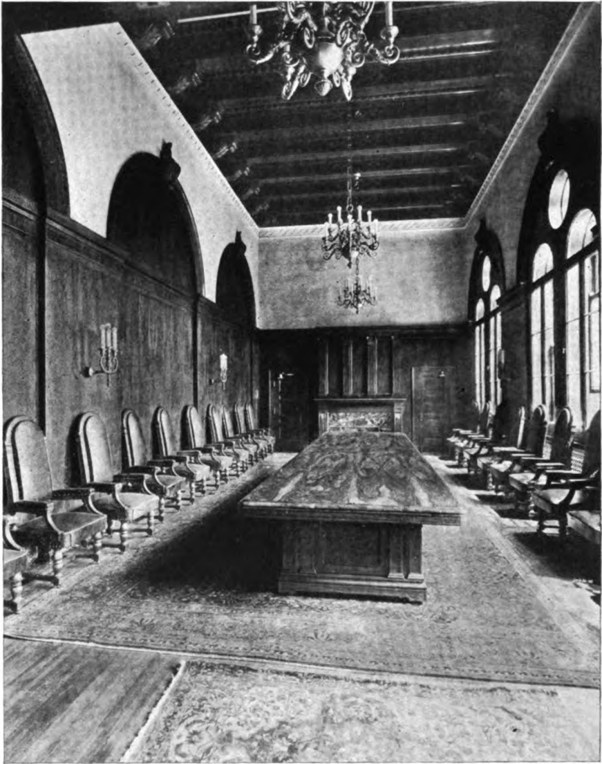
Where the Directors Meet. A well-lighted, well-furnished room.
