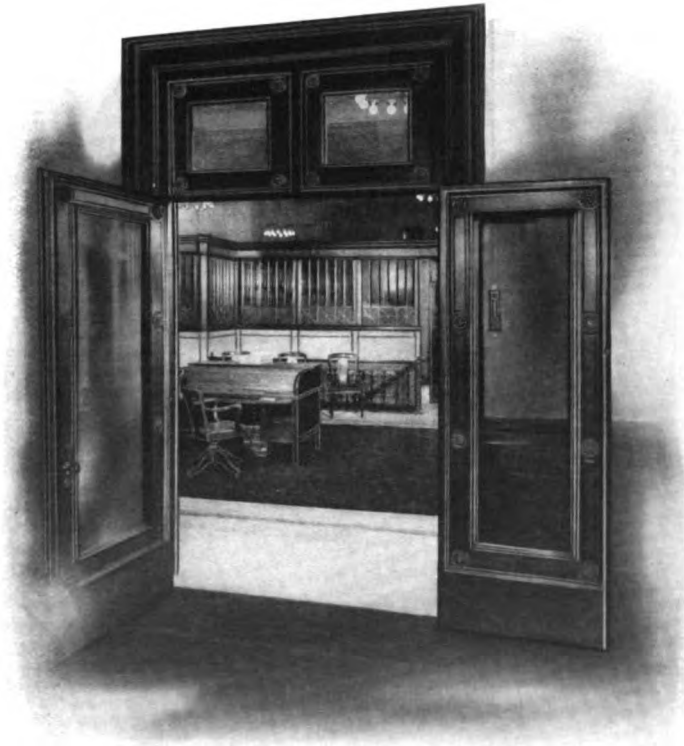
View from the President's Office across Reception Room into Main Banking Room
