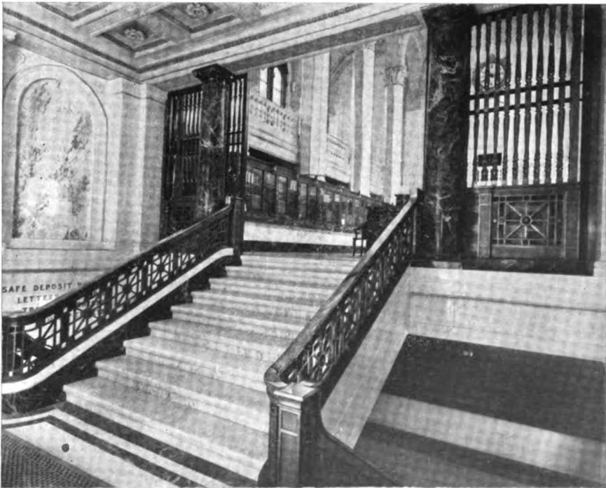
A Glimpse of the Main Banking Room as seen from the Vestibule. At the extreme left the stair turns down to the Safe Deposit Vaults.
