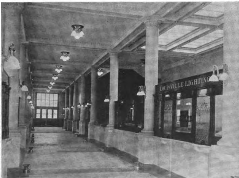
Offices of Louisville (Ky.) Lighting Company.—An Attractively Lighted Corridor. Showing Combination of Globes and Bell-Shaped Reflectors.
