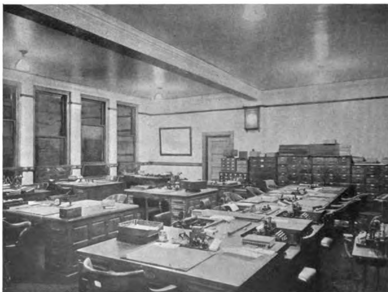
Section of Carnegie Steel Company's Offices, Pittsburg, Pa.—Correct Desk Lighting Effected by Holophane Shades Placed on the Ceiling, Giving a Uniform Light Distribution on Desk Tops, Causing Locally Arranged Desk-Lighting Units to be Unnecessary.
