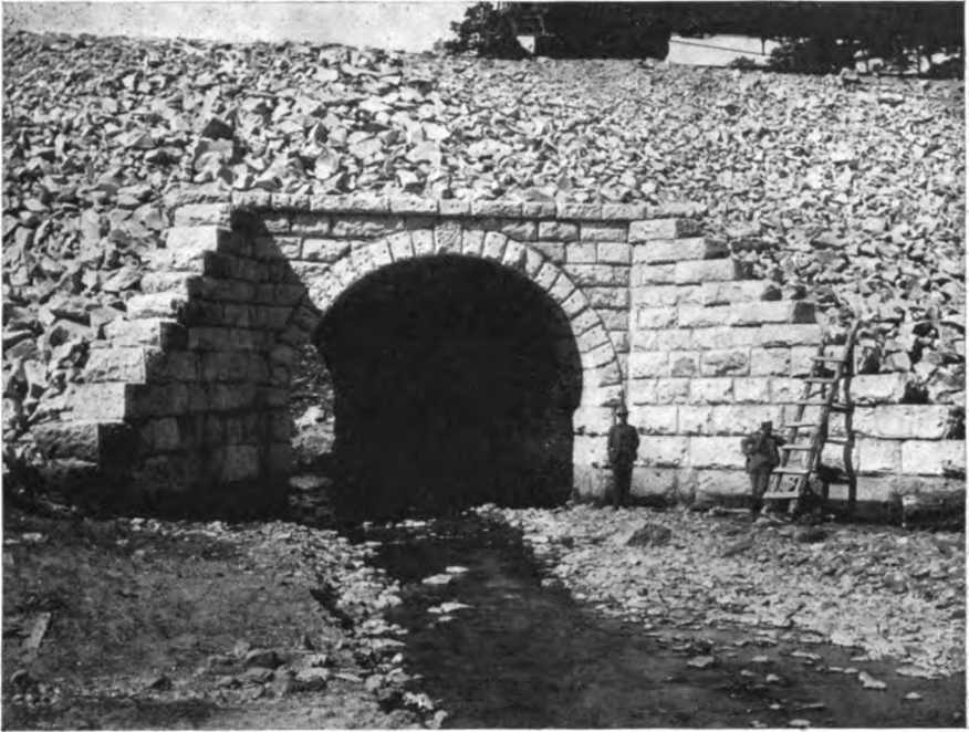
Stone Arch Culvert 6.00 Meter, at Kilometer 77 State of Chihuahua, Mexico.
