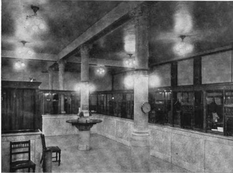
Merchants' Bank, Rochester, N. Y.—An Effective Method of Grouping Lamps in Alabaster Globes.
