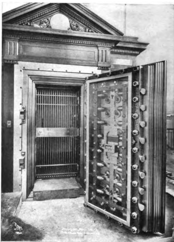
Entrance and Door to One of the Vaults
