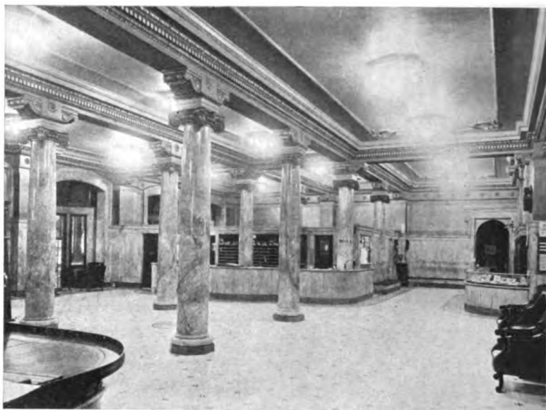
Lobby Hotel Iroquois, Buffa'o, N. Y.—Ceiling Fixtures Combining Glass Beading Shades With a Cluster of Unshaded Bulbs. This Style is Well Adapted to Bank Lighting.
