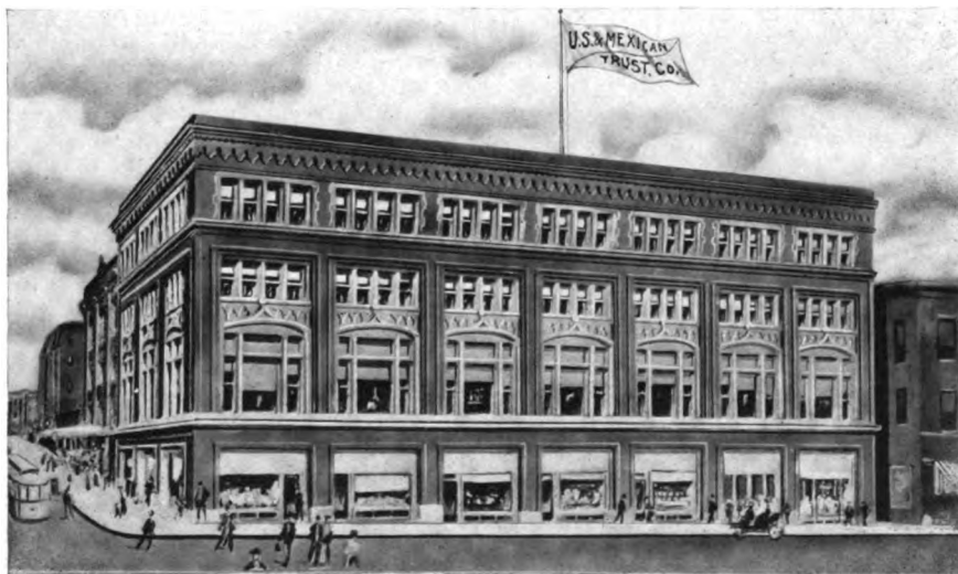
United States and Mexican Trust Co. Building, Kansas City, Mo. The General Offices of the Kansas City, Mexico and Orient Railway.
