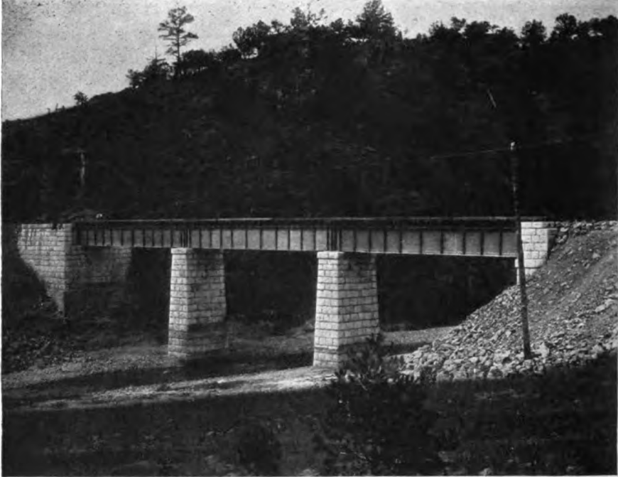
Bridge across the Pichachic Arroyo.
