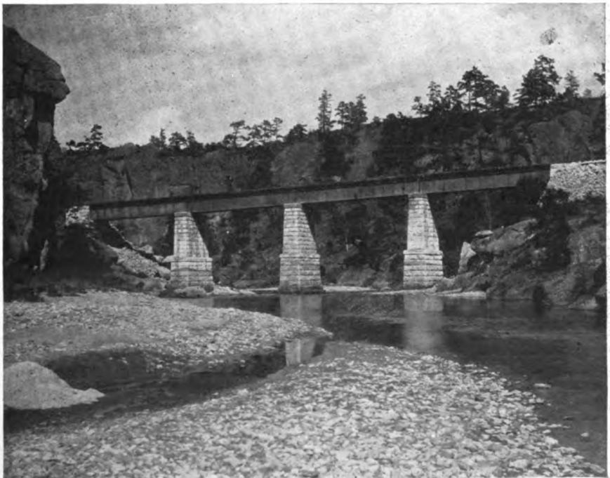
Steel Bridge across Guerrero River.
