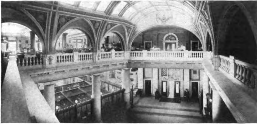
A View from the Mezzanine Floor. The National Bank of Commerce, St. Louis.
