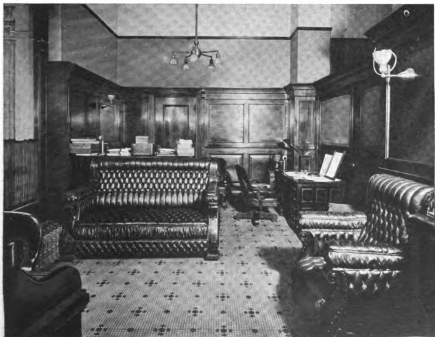
Private Office of Mr. Carpenter and Mr. Baggot.
