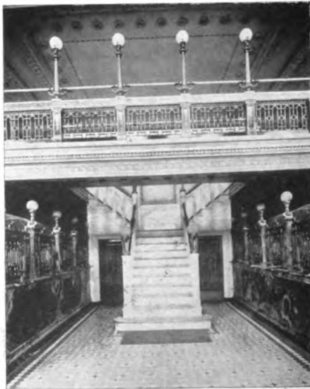
Staircase Leading to the Mezzanine Floor.
