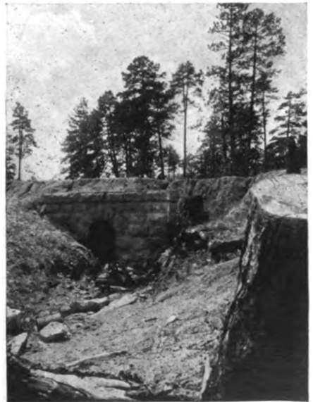
Stone Culvert, Kilometer 57.
