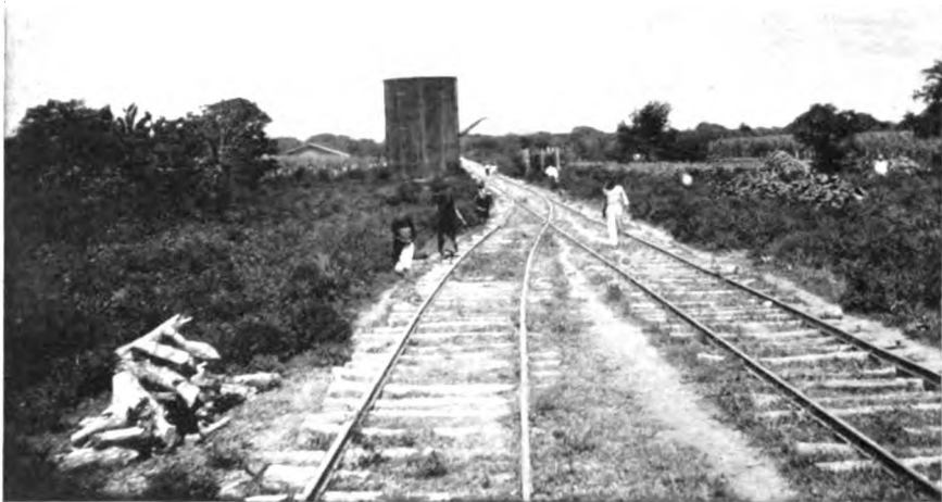
A Section of the Roadbed.
