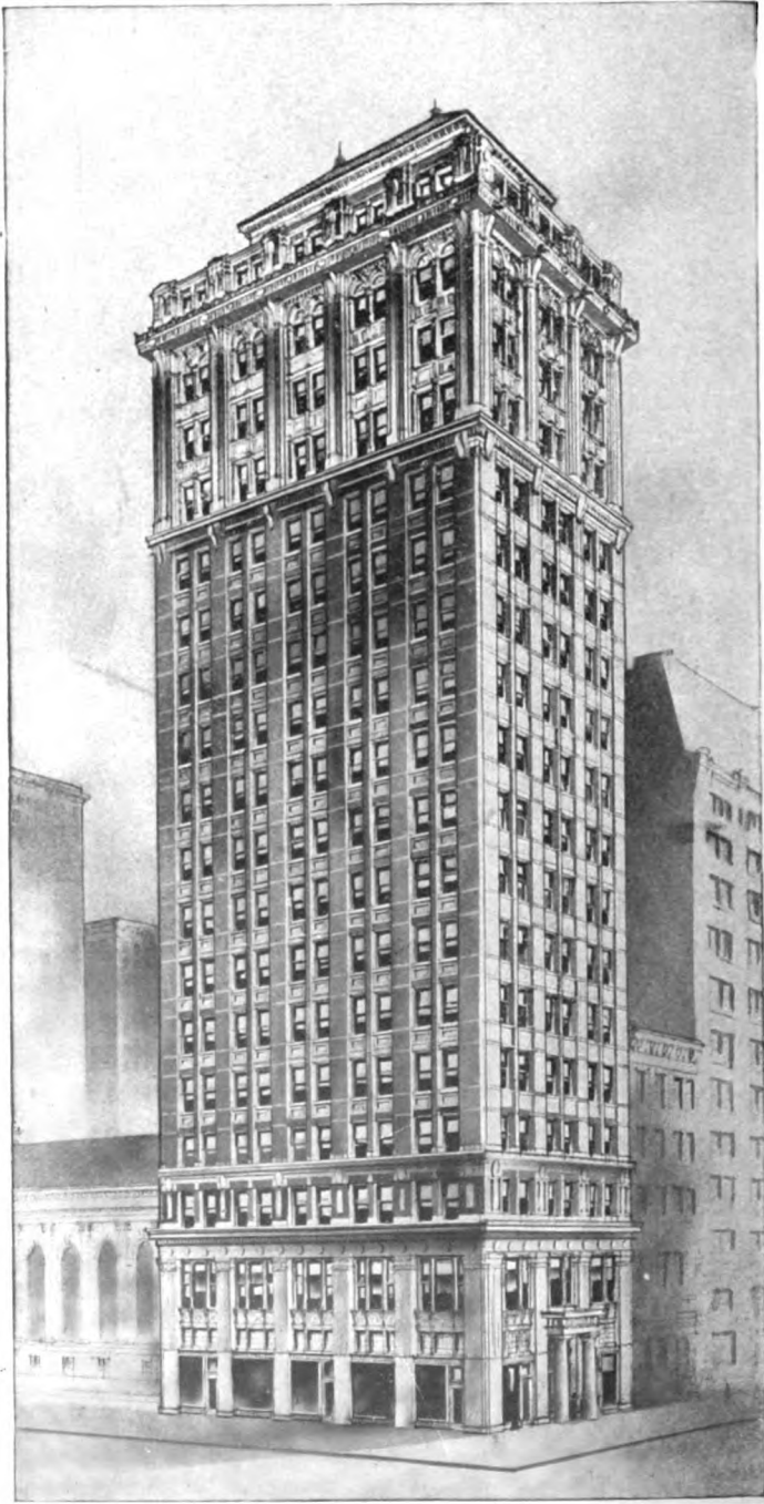
NEW UNDERWOOD BUILDING, NEW YORK CITY
