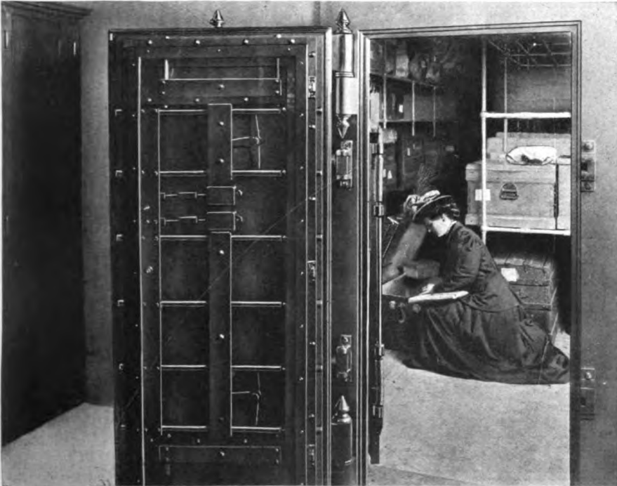
ONE OF THE STORAGE VAULTS FOR TRUNKS AND BULKY PACKAGES
