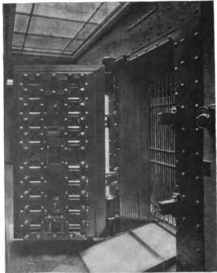
VAULT DOOR, SAFE DEPOSIT VAULT, WASHINGTON TRUST CO.
