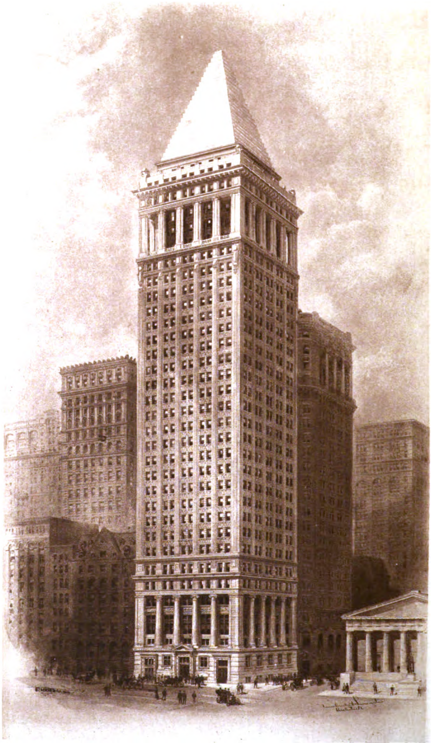
BANKERS TRUST COMPANY BUILDING WALL AND NASSAU STREETS NEW YORK
