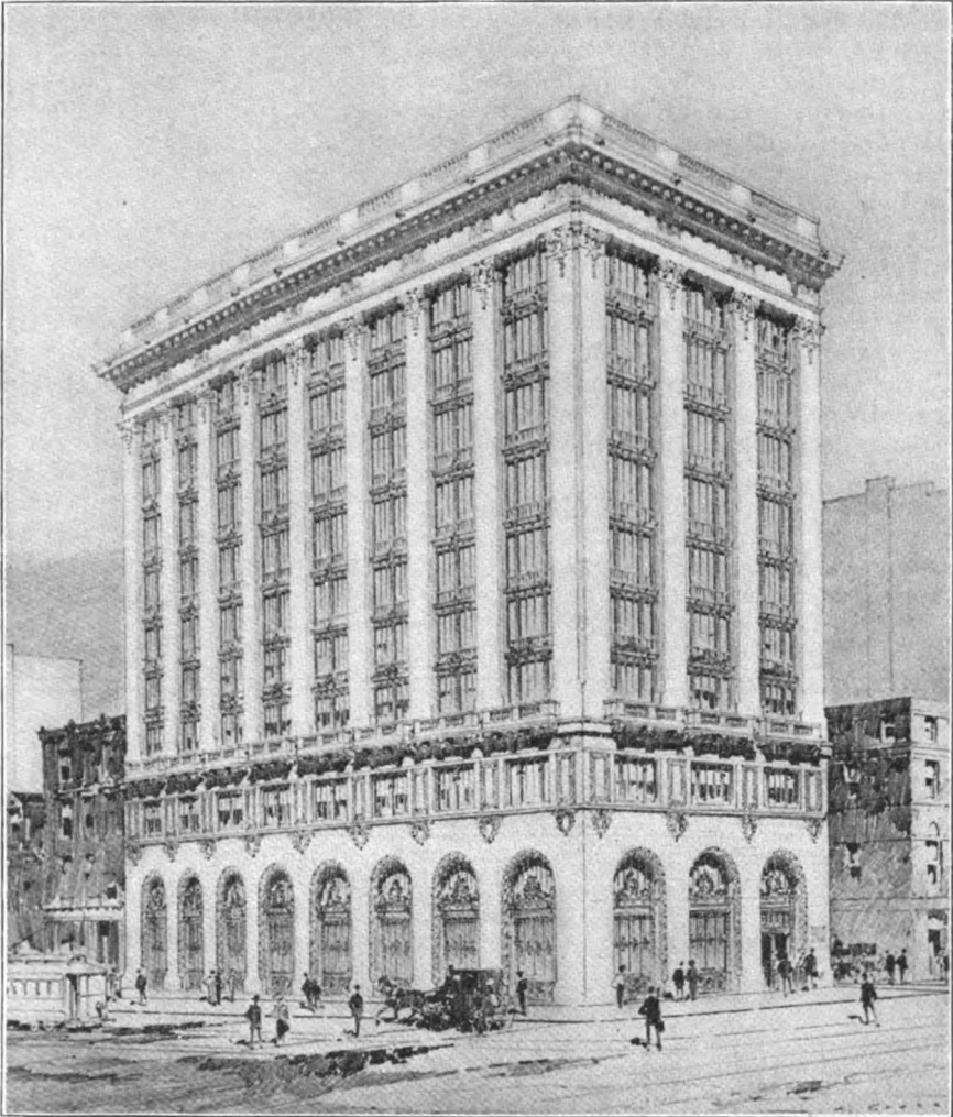
NEW BUILDING NOW UNDER CONSTRUCTION FOR THE MERCHANTS NATIONAL BANK, BOSTON
