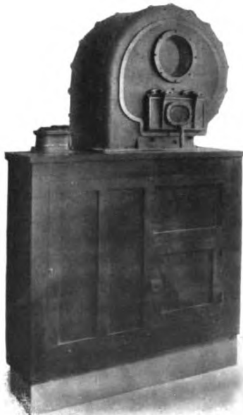
ONE OF THE TWENTY STATIONS IN THE PNEUMATIC TUBE SYSTEM, BANKERS TRUST COMPANY BUILDING, NEW YORK
