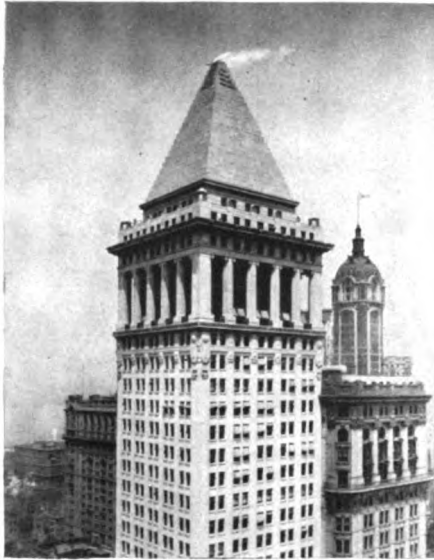
TWENTY UPPER STORIES AND THE NINETY-FOUR FOOT PYRAMID SURMOUNTING THE FORTY-ONE STORY BANKERS TRUST COMPANY BUILDING. SINGER TOWER IN BACKGROUND.
