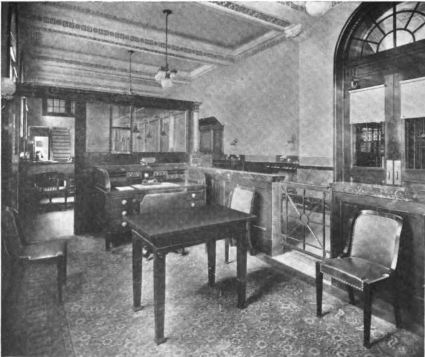
CASHIER'S OFFICE, NEW HAMPSHIRE NATIONAL BANK, PORTSMOUTH
