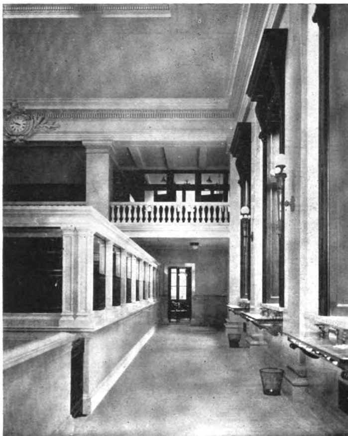
BARNETT NATIONAL BANK, JACKSONVILLE, FLA. EASTERN LOBBY, LOOKING NORTH.
