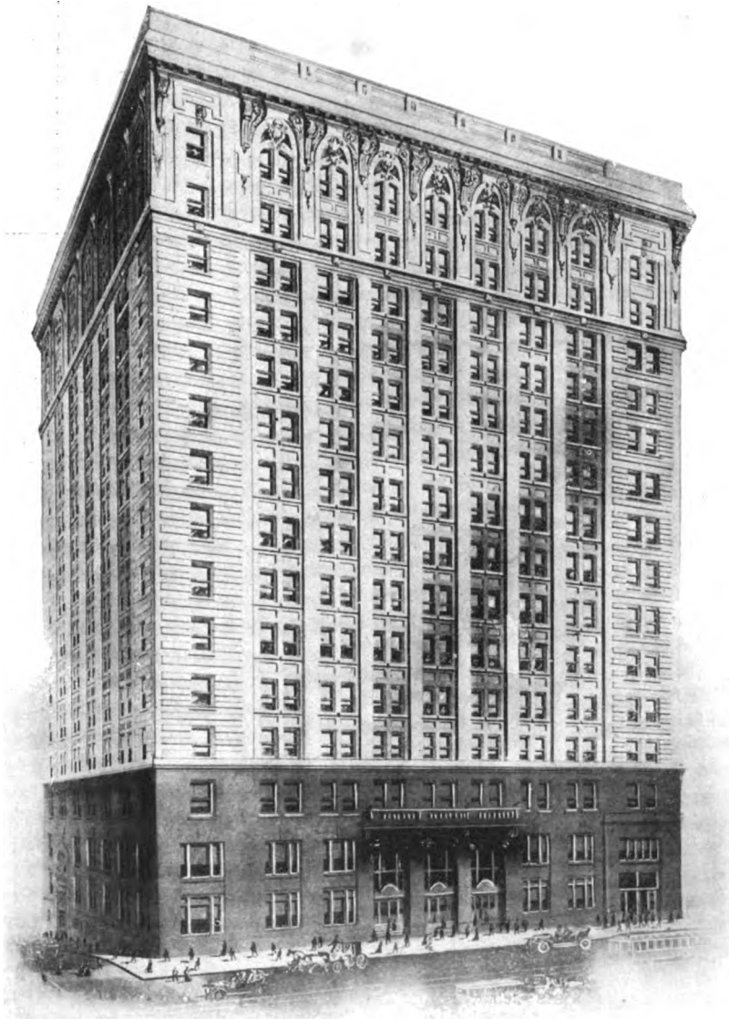
BUILDING OF THE SOUTHWEST NATIONAL BANK OF COMMERCE, KANSAS CITY, MO.
