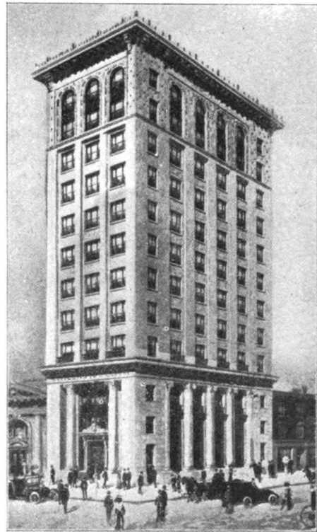
NEW BANK AND OFFICE BUILDING IN COURSE OF CONSTRUCTION FOR THE CITIZENS NATIONAL BANK, RALEIGH, N. C.
