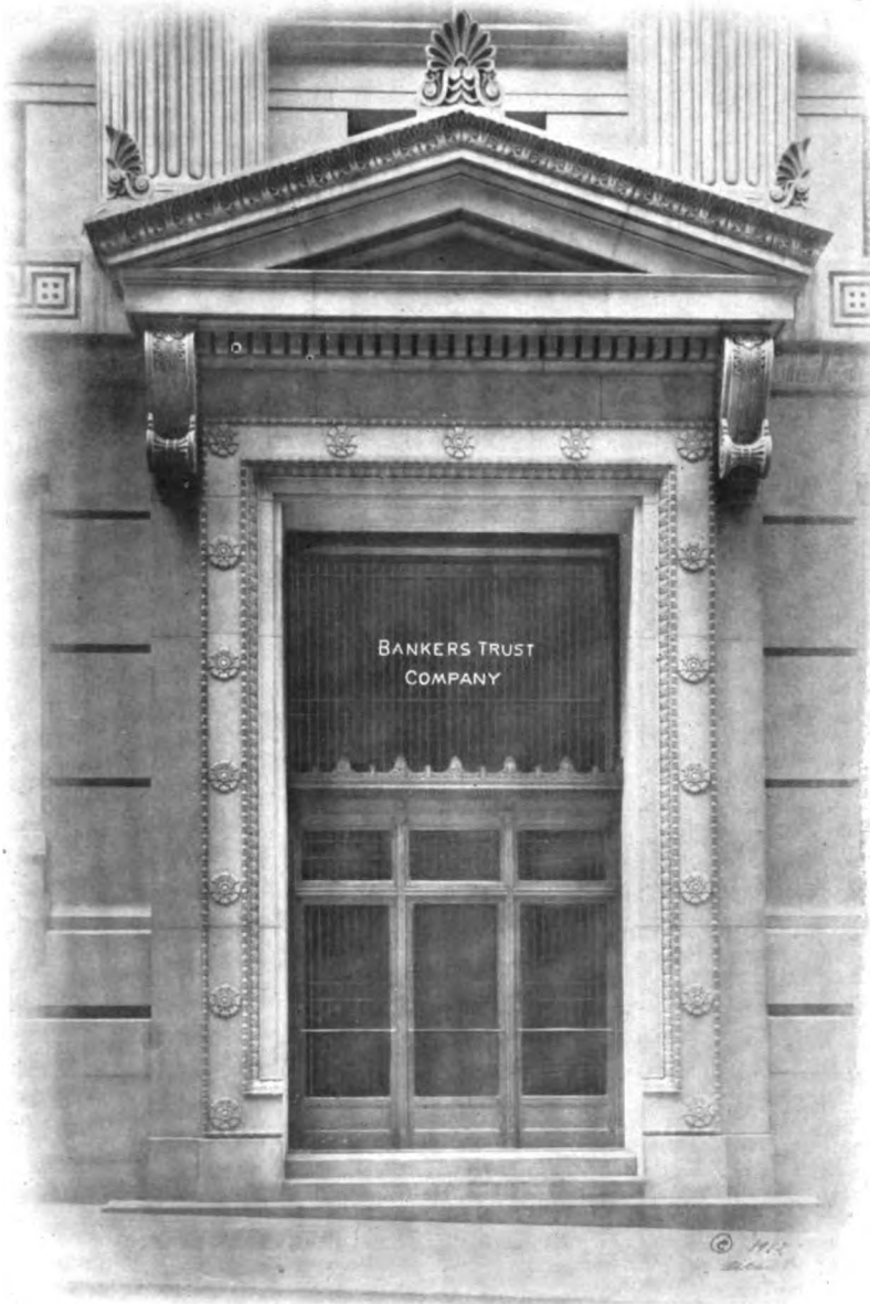
WALL STREET ENTRANCE OF THE BANKERS TRUST COMPANY BUILDING, NEW YORK
