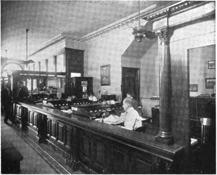
MERCHANTS NATIONAL BANK, RICHMOND—PORTION OF OFFICERS' QUARTERS
