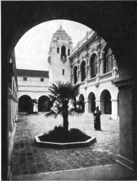
PATIO, SOUTHERN CALIFORNIA; COUNTIES BUILDING
