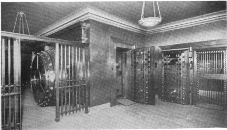
SAFE DEPOSIT, CASH AND RECORD VAULTS THE SAN DIEGO SAVINGS BANK, SAN DIEGO, CAL.
