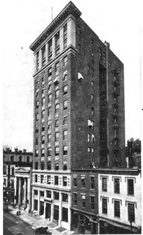
TRAVELERS BUILDING—VIRGINIA TRUST COMPANY OCCUPIES A PORTION OF GROUND FLOOR
