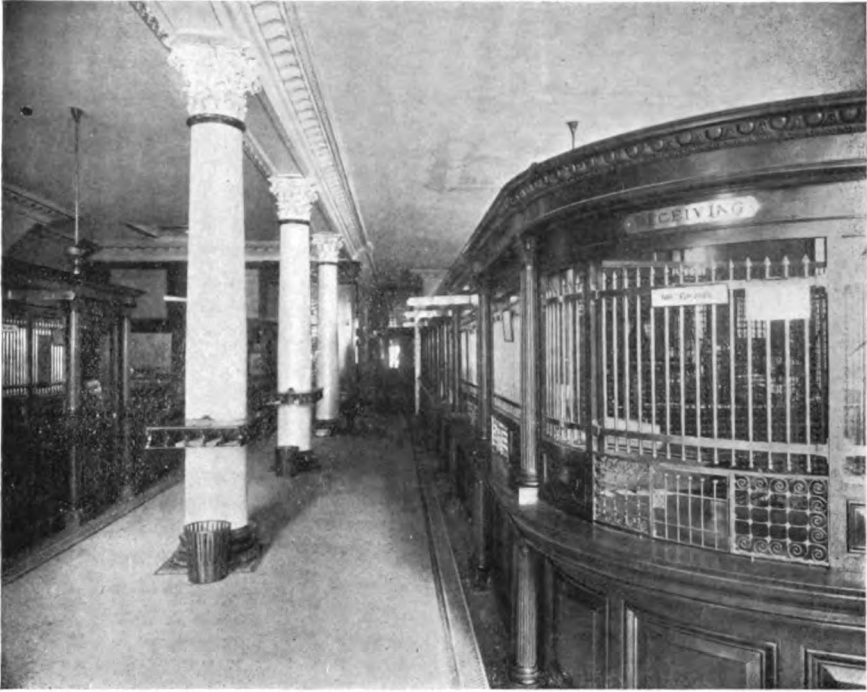
MAIN BANKING ROOM, MERCHANTS NATIONAL BANK, RICHMOND
