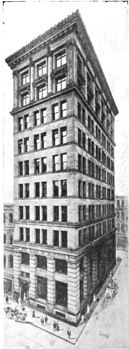
MONTREAL BRANCH THE BANK OF OTTAWA, OTTAWA, ONTARIO
