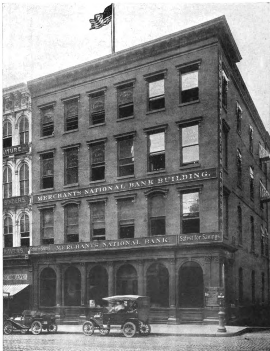
MERCHANTS NATIONAL BANK BUILDING, RICHMOND
