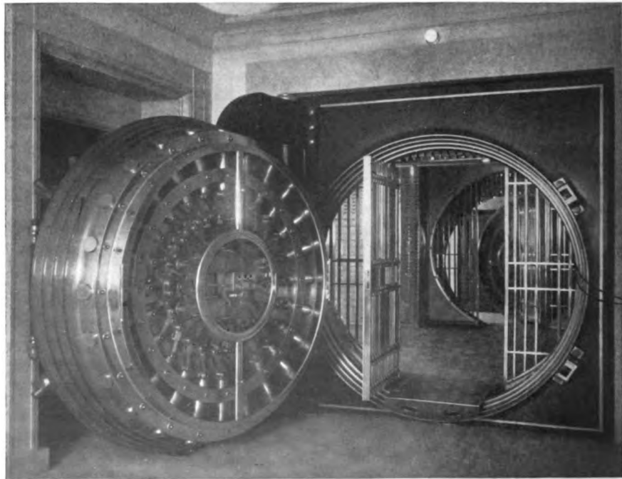
VAULT DOOR THE MARINE NATIONAL BANK, BUFFALO, N. Y.
