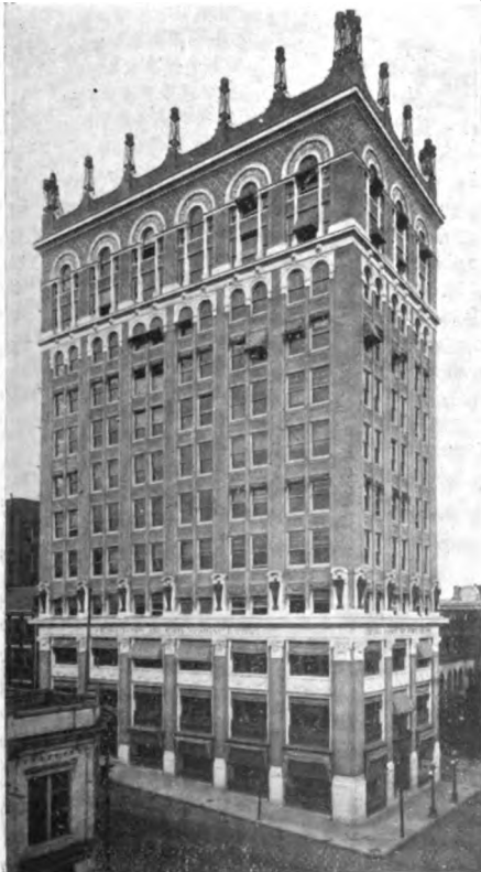
VIRGINIA RAILWAY AND POWER BUILDING
