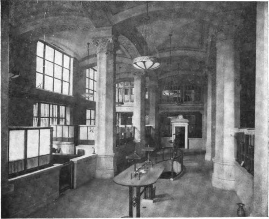
THE LOBBY LOOKING TOWARD REAR FIRST NATIONAL BANK, RICHMOND, VA.
