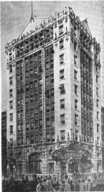
NEW BUILDING IN COURSE OF CONSTRUCTION FOR THE NATIONAL BANK OF WEST VIRGINIA, AT WHEELING
