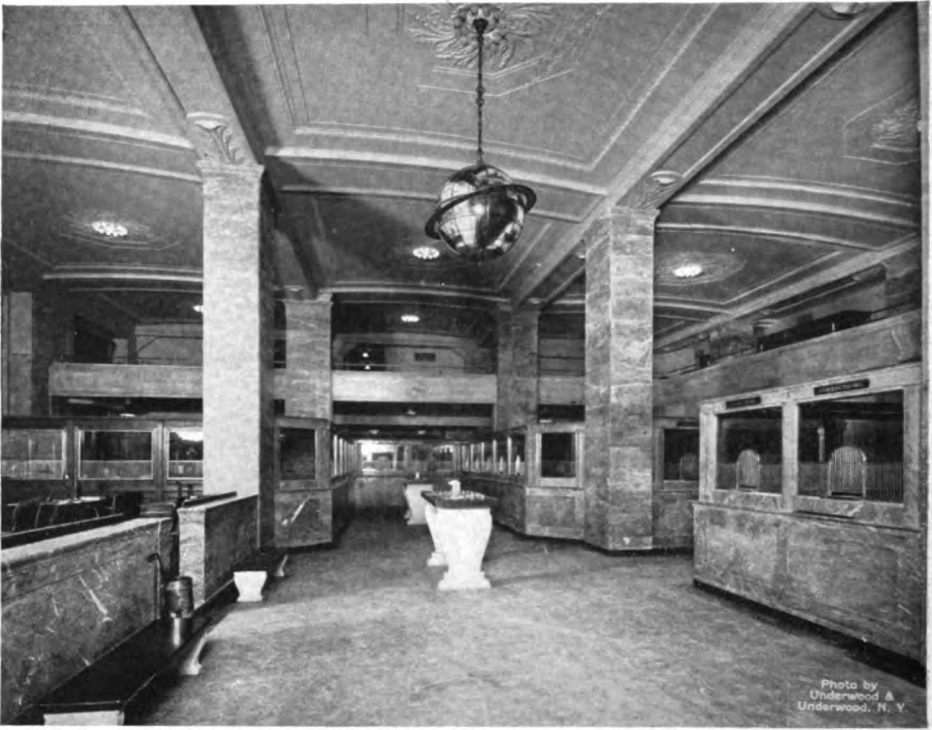
INTERIOR, LOOKING DOWN THE LOBBY FROM FRONT DOOR
