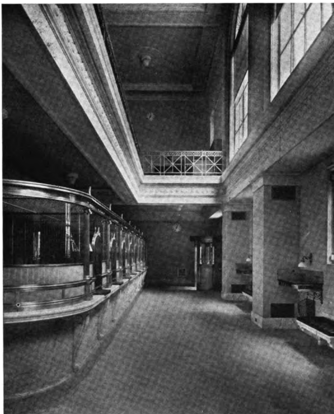
VIEW OF MAIN BANKING ROOM THE NEW HAVEN BANK, N. B. A., NEW HAVEN, CONN.
