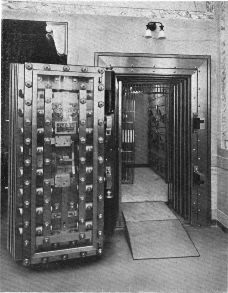
CURRENCY AND SECURITY VAULT SHOWING MASSIVE STEEL DOOR FIRST NATIONAL BANK, SYRACUSE, N. Y.
