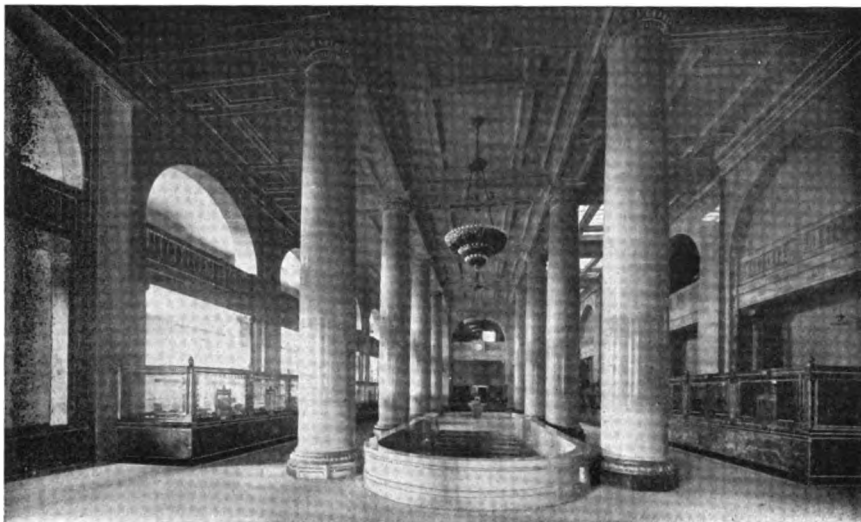
MAIN BANKING ROOM FROM CASHIER'S DESK
