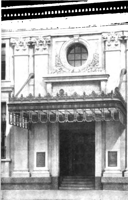
MAIN ENTRANCE TO THE BUILDING
