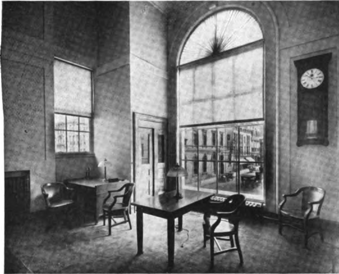
COMMITTEE ROOM AND LIBRARY ON MEZZANINE FLOOR THE NEW HAVEN BANK, N. B. A., NEW HAVEN, CONN.
