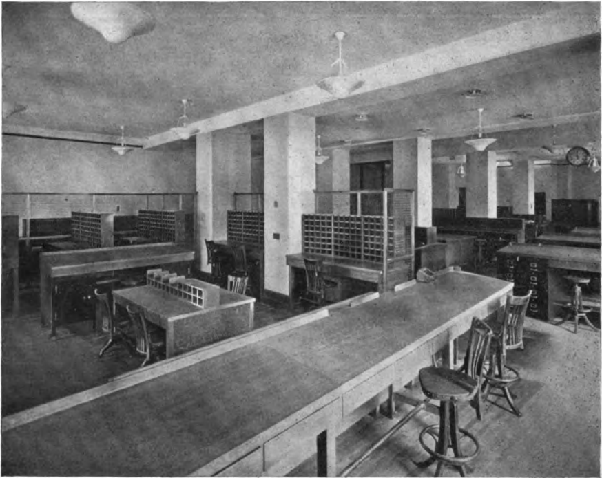
CHECK DESKS, AMERICAN EXCHANGE NATIONAL BANK, NEW YORK
