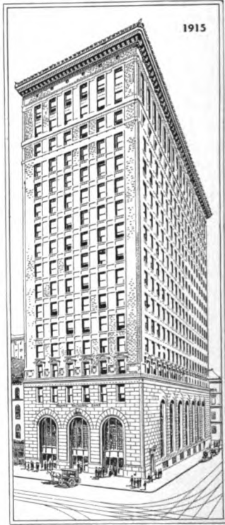
METSEY STONE AND TERRA COTTA FIRE-PROOF BUILDING OF THE MARINE NATIONAL BANK. THE BANKING ROOMS, YOU SEE, ARE THE FIRST IN THE WORLD'S VAULTS IN THE FIRST BUILDING.
