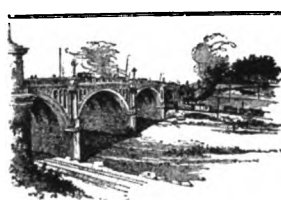
The great North Broadway reinforced concrete bridge over the Los Angeles River—a representative type of bridge construction in Southern California.
