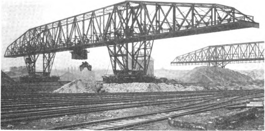
View of Traveling Cranes or "Ore Bridges" in Bethlehem Steel Company's storage yard
