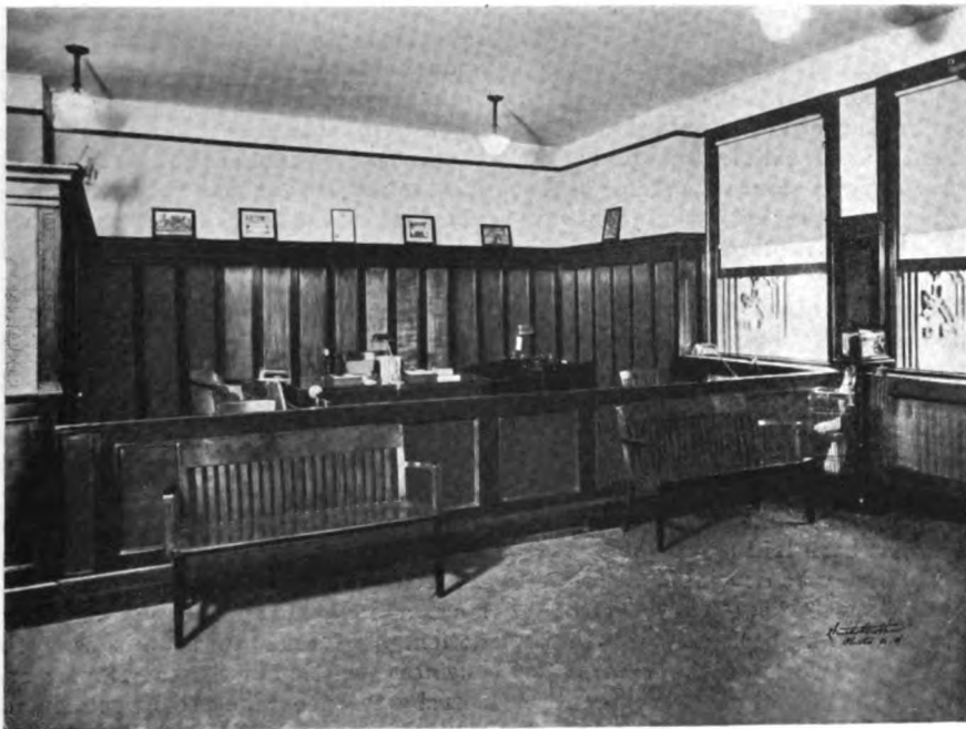
Manager's Office, Philippine National Bank, New York Agency
