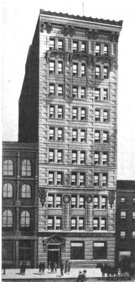
Montreal Branch, Union Bank of Canada
