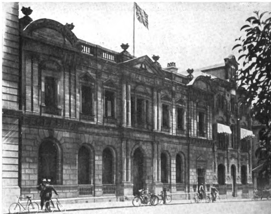
National Bank of South Africa, Limited, Head Office, Pretoria
