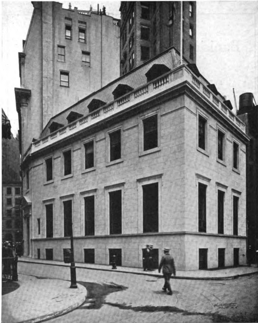
The New Addition to the Offices of Brown Brothers & Co., at 4 and 5 Hanover Street
