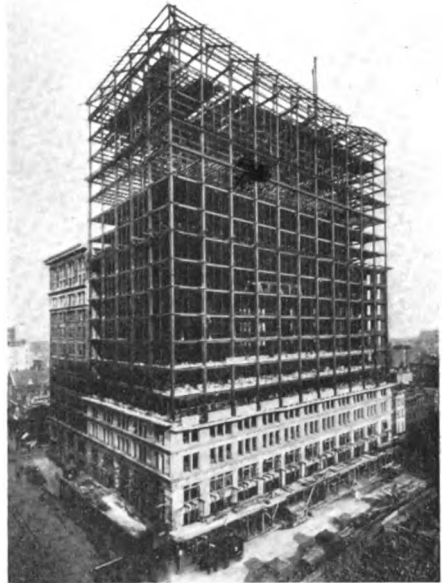
Modern Sky-Scraper, showing Bethlehem Grey Beams
