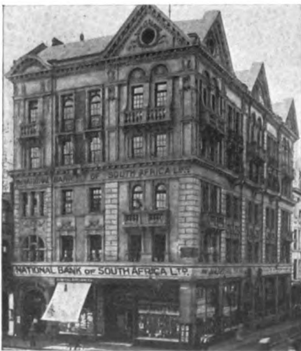
National Bank of South Africa, Ltd., Pritchard Street Branch, Johannesburg
