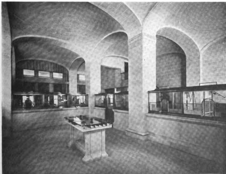
Main Banking Room and public space from Broadway entrance
