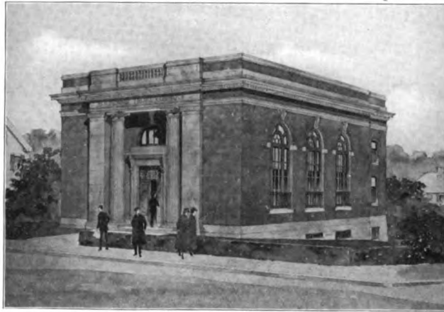
MODERN BANK BUILDING NOW UNDER CONSTRUCTION FOR THE ROCKLAND TRUST CO., ROCKLAND, MASS.
